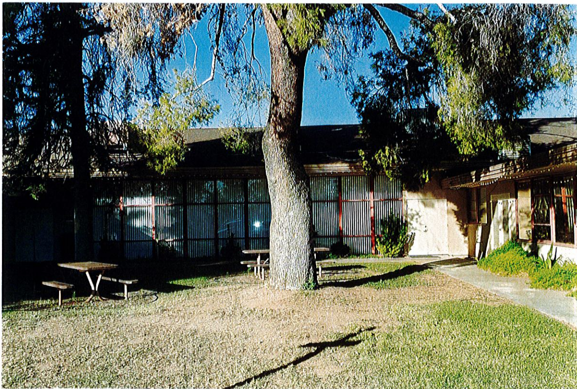
Photo OS3: East side of original sanctuary. Note large steel casement windows and that floor is not elevated much above the lawn area (typical for 1950s construction).
