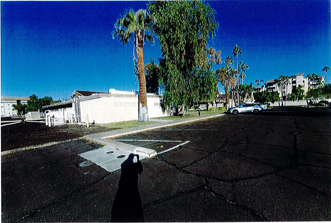
Photo OS4: Southeast corner of kitchen/classroom wing. Note small windows mounted high and plain walls. Utility access to campus is along the south wall to the left.
