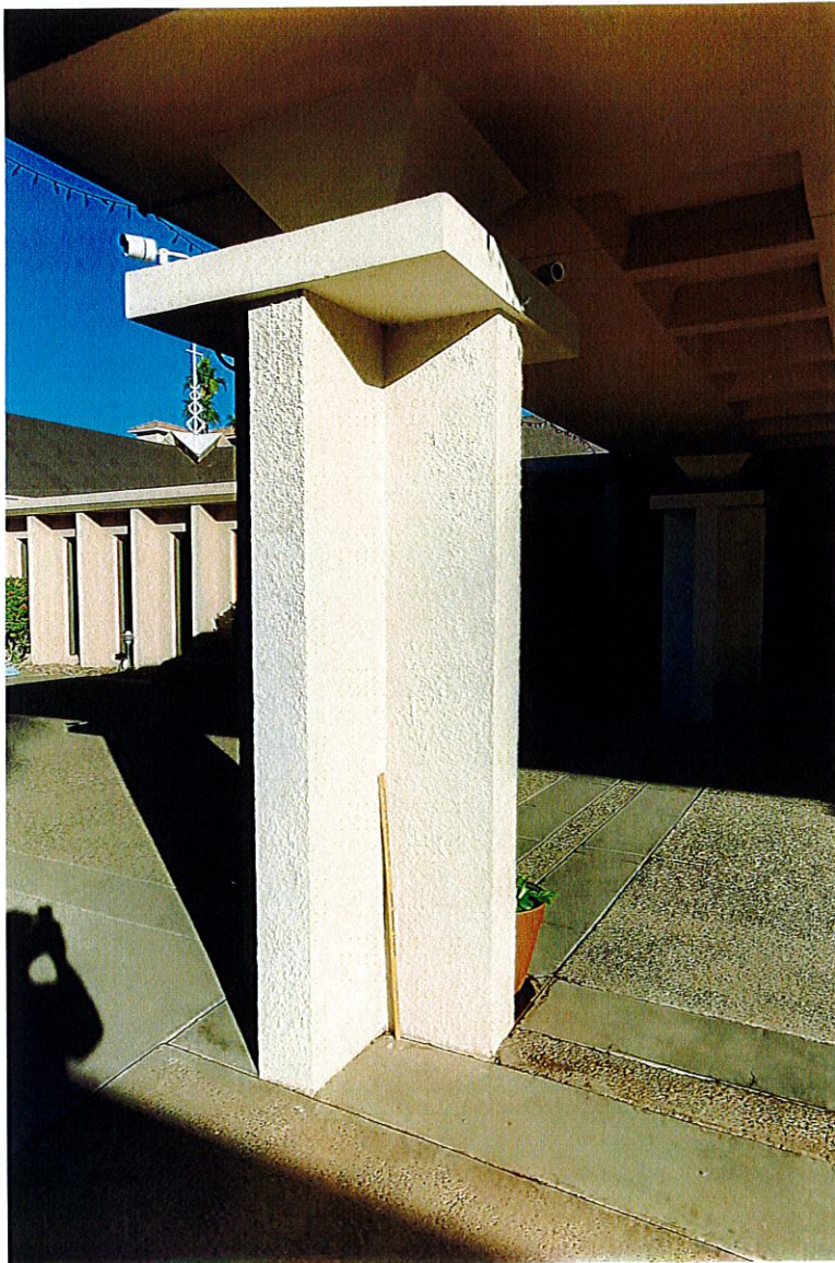
Photo NS10: Column detail at the entry ramada. The exposed aggregate pavement was common in the 1960s and 1970s.
