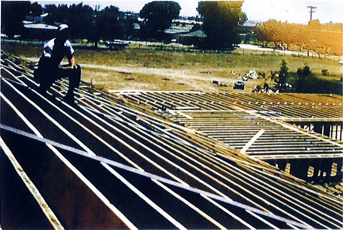
Photo H6: Construction on the roof of the new sanctuary in 1965, looking eastward. Note homes across Miller Road and intersection with Indian School Rd. on the right.
