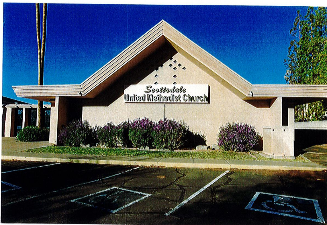
Photo NS3: The east end of the new sanctuary.
