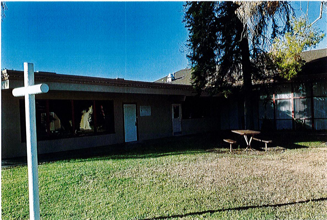
Photo OS5: North side of the kitchen/classroom wing. Steel casement windows matching the office wing were installed.
