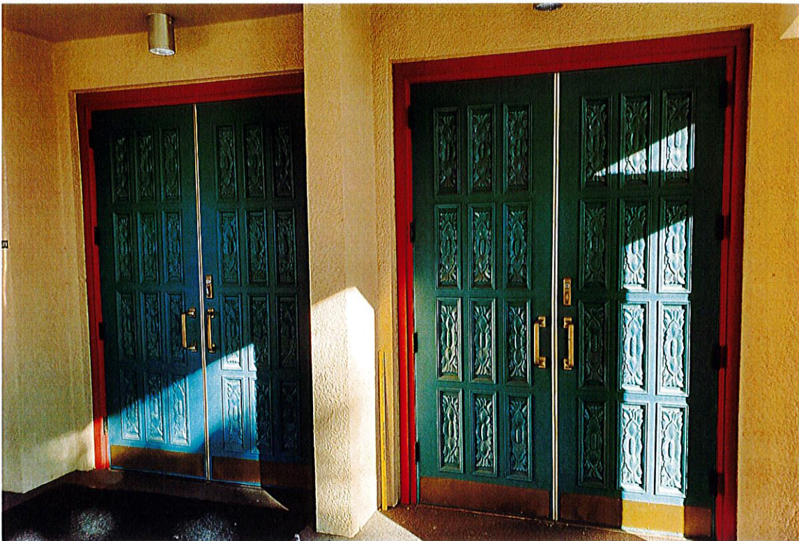
Photo NS12: The exterior entrance doors. These were hand carved on special order from the Tucson area.
