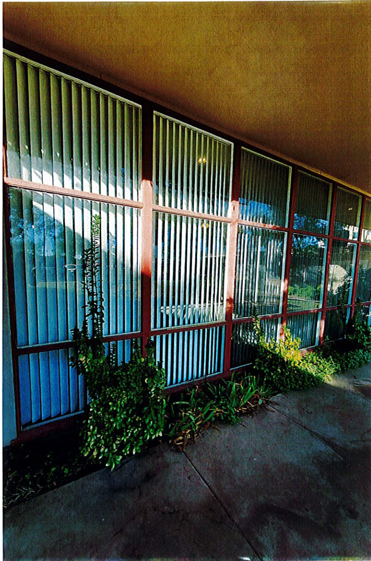
Photo OS8: Close-up of steel case windows on the east side of the original sanctuary. These panels were not operable.
