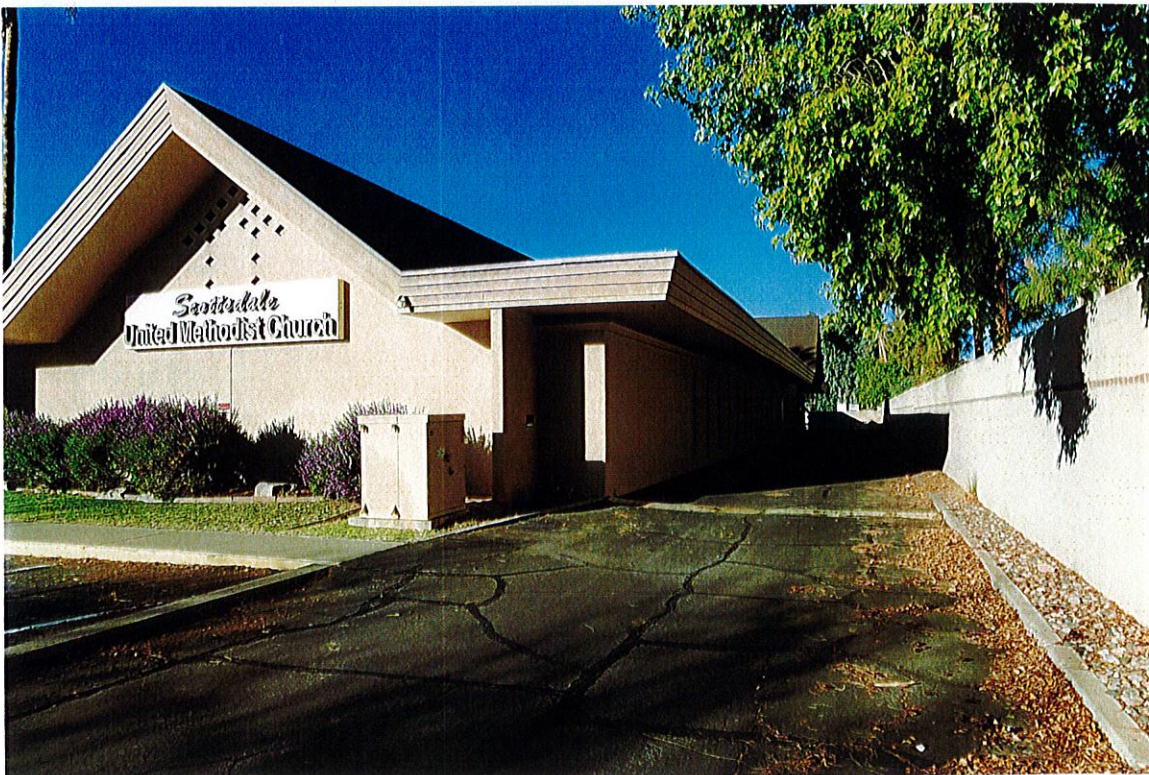
Photo NS2: The northeast corner of the new sanctuary looking along the north wall.
