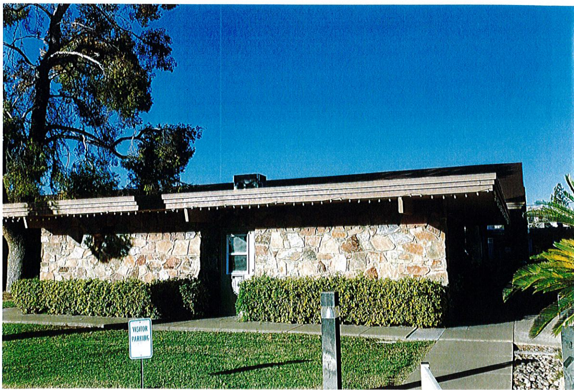
Photo OS1: Northeast corner of the office wing. Note the flagstone veneer and the canted eave detail.
