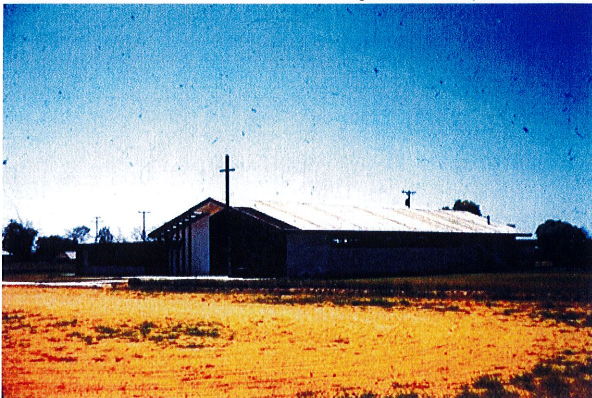
Photo H3: The newly constructed church buildings ca 1956 looking southeast. Note single family homes on the property across Miller Road on the left. The Song home was under the trees behind the right end of the sanctuary building. Parking was on the dirt lot.
