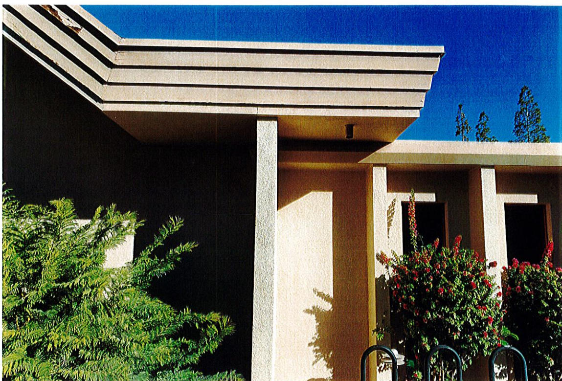
Photo NS37: Roof eave details where the chapel roof meets the restroom/foyer part of the building.
