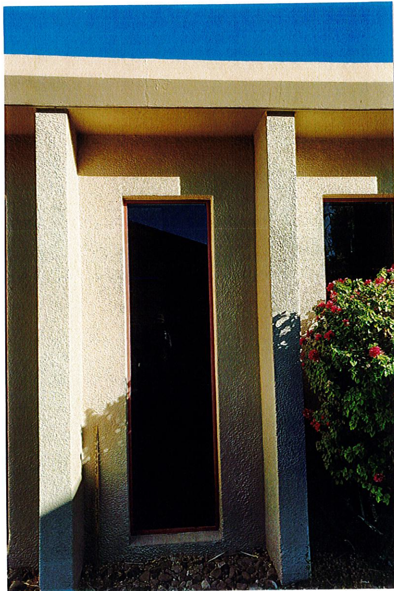
Photo NS13: Along a hallway on the south side of the new sanctuary building the exterior wall is composed of a rhythm of narrow windows placed in 'shadow boxes' between 'buttress' walls that project for the main wall. This reduces sun exposure on the windows in the summer months.
