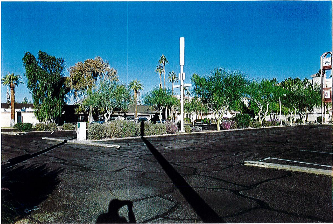
Photo S2: View from southeast corner looking northwest. Note the cell tower on top of parking area light pole.
