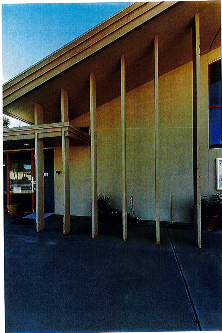
Photo OS15: Close-up of vertical wood slat columns on north side of sanctuary. These visually tie the sanctuary and office wings roofs together.
