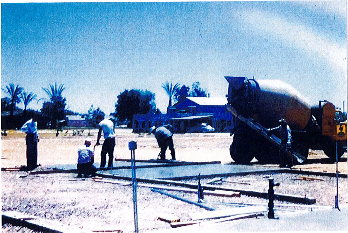
Photo H13: Construction on new education wing west of the first sanctuary building (ca 1959). Note Ascension Lutheran Church in background on the right. (looking southwest)
