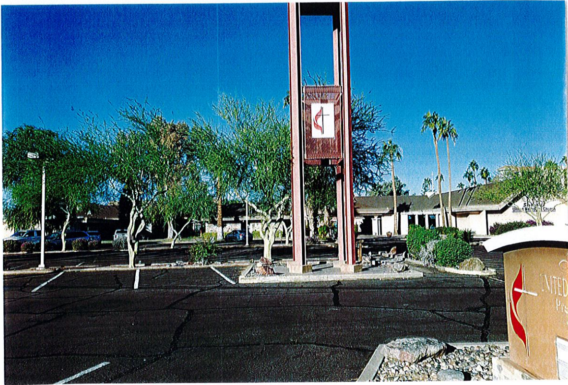
Photo S3: Photo from the center of parcel on the east side looking west (just south of main entry off of Miller Road).
