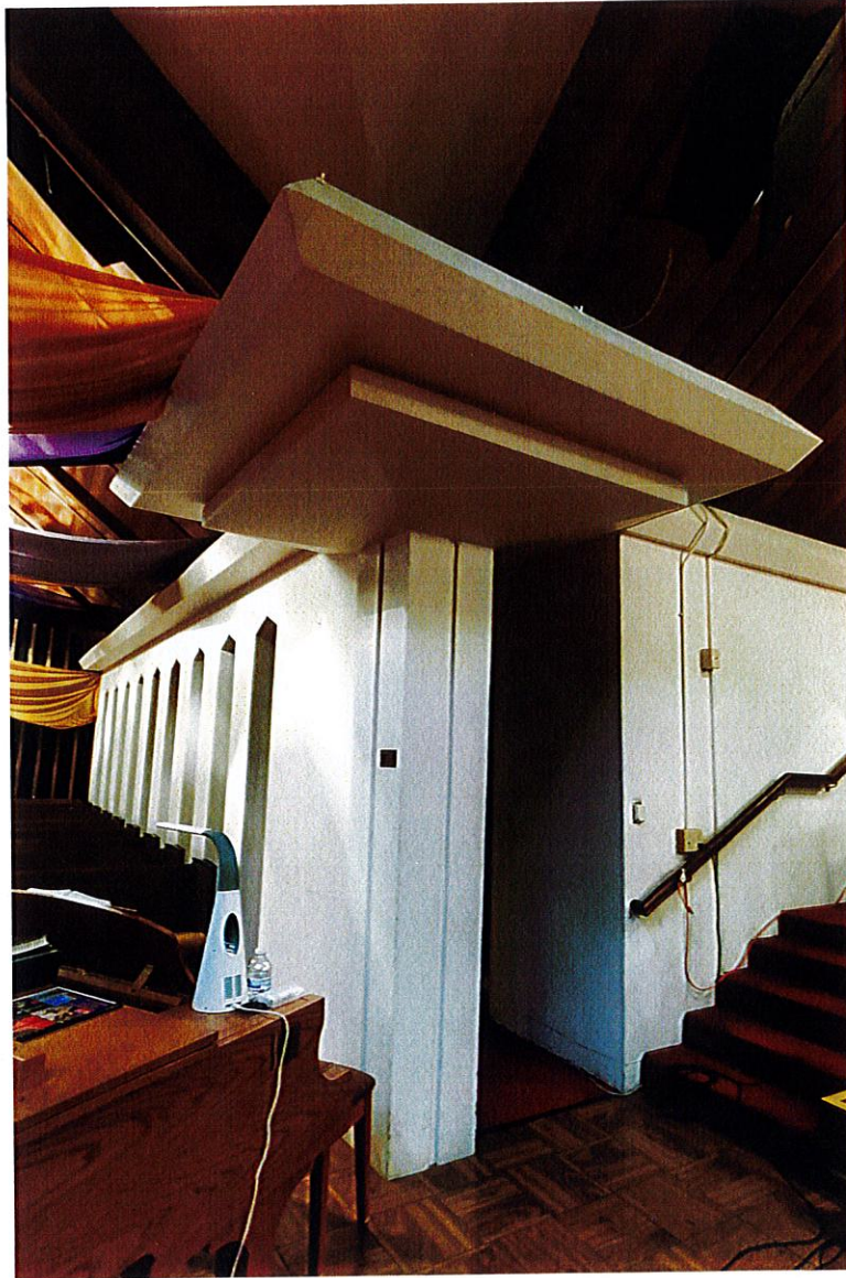
Photo NS24: Corner column detail where chapel and main sanctuary spaces meet at pulpit/dais area. The 'V' shaped projection runs along the top of the walls and columns around the interior spaces. Notice single flute in center of column.
