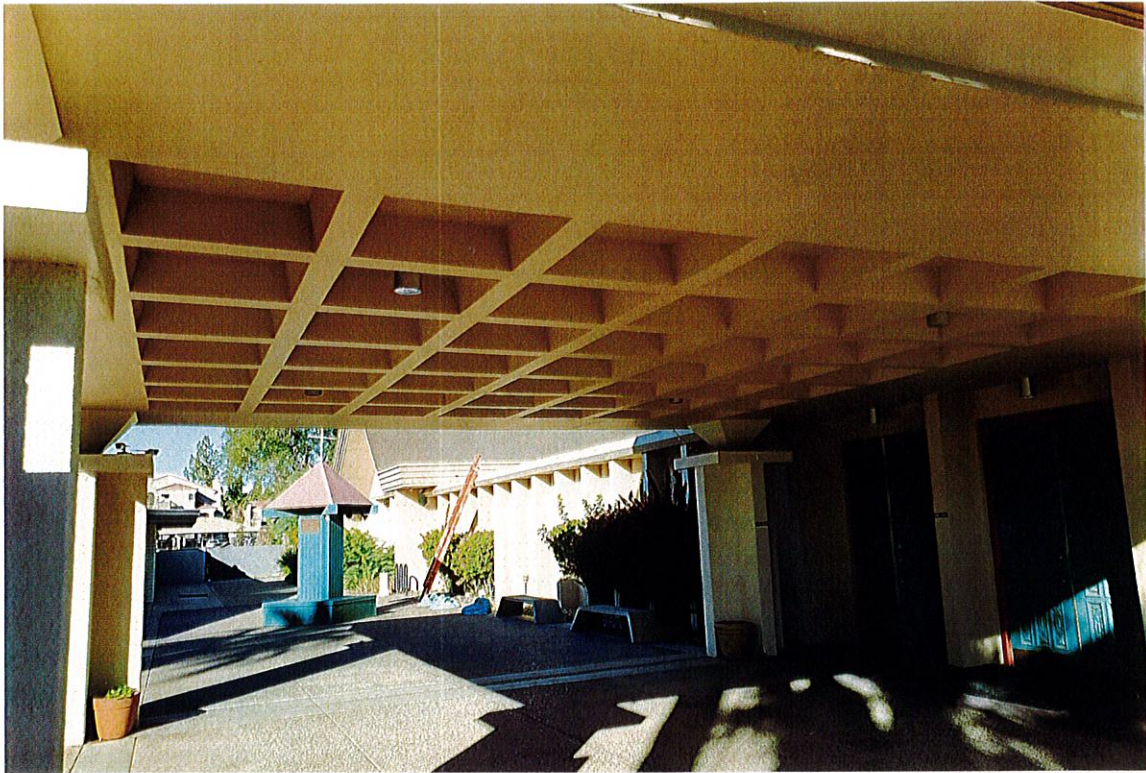
Photo NS11: Close-up of ceiling of entrance ramada. The “waffle” type concrete roof structure was common in the early to mid-1960s.
