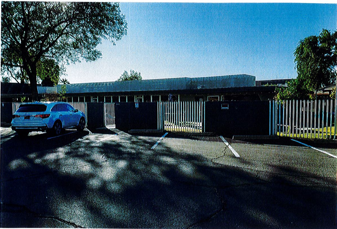
Photo E2: This photograph shows the façade on the north side of the new education building. Note the larger windows on this side than on the southern side. The fence for the play area is also more substantial.
