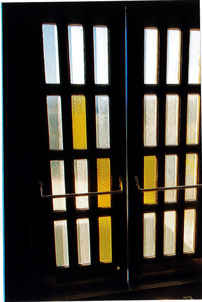
Photo NS21: The exterior entrance doors in the southwest quadrant that lead to the chapel worship space. These are similar in construction to the interior entrance doors to the main sanctuary space.
