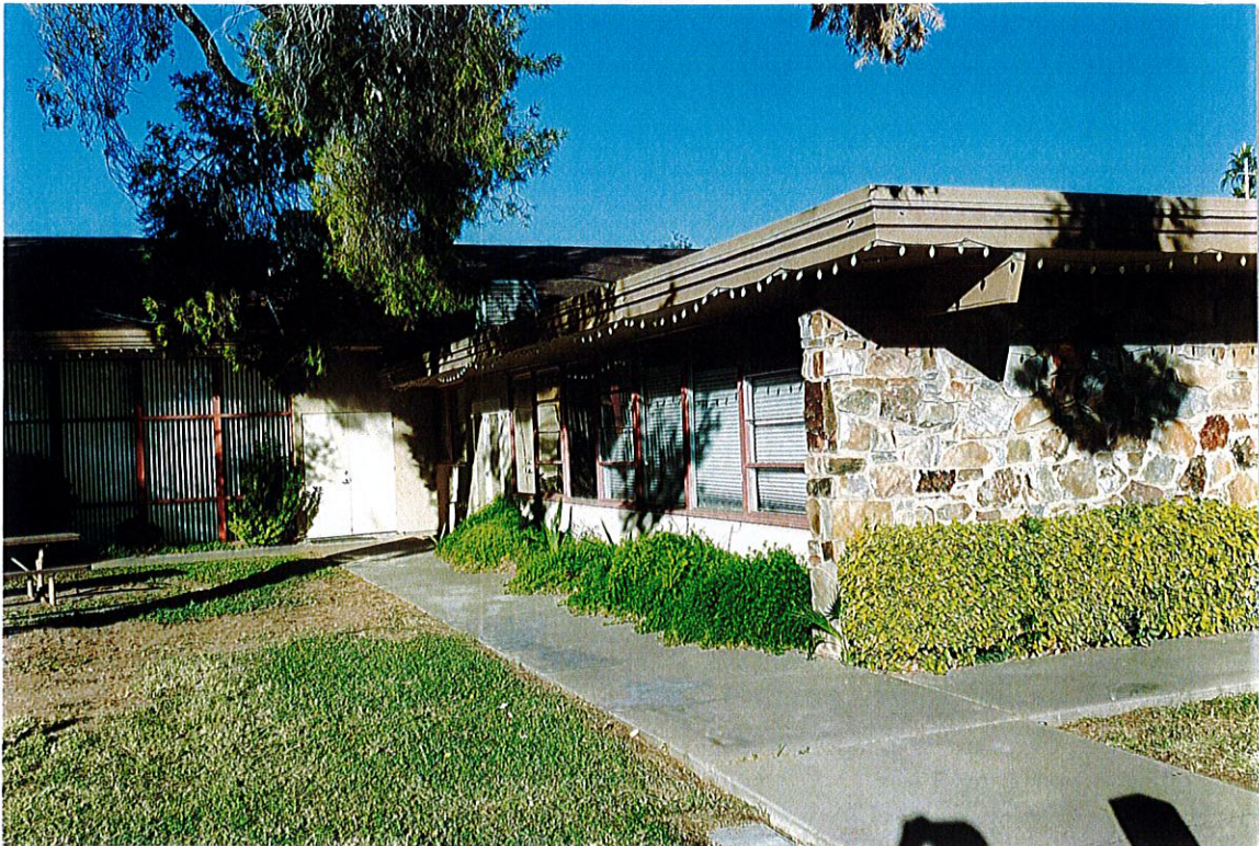
Photo OS2: Southeast corner of office wing. Note the stone veneer and steel casement windows. Side entrance to original sanctuary at corner.
