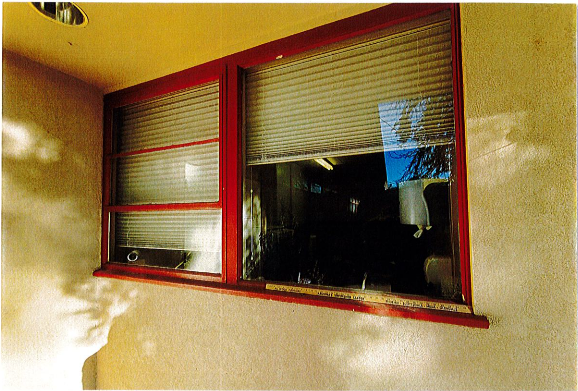
Photo OS9: Steel casement windows at southwest corner of office wing.
