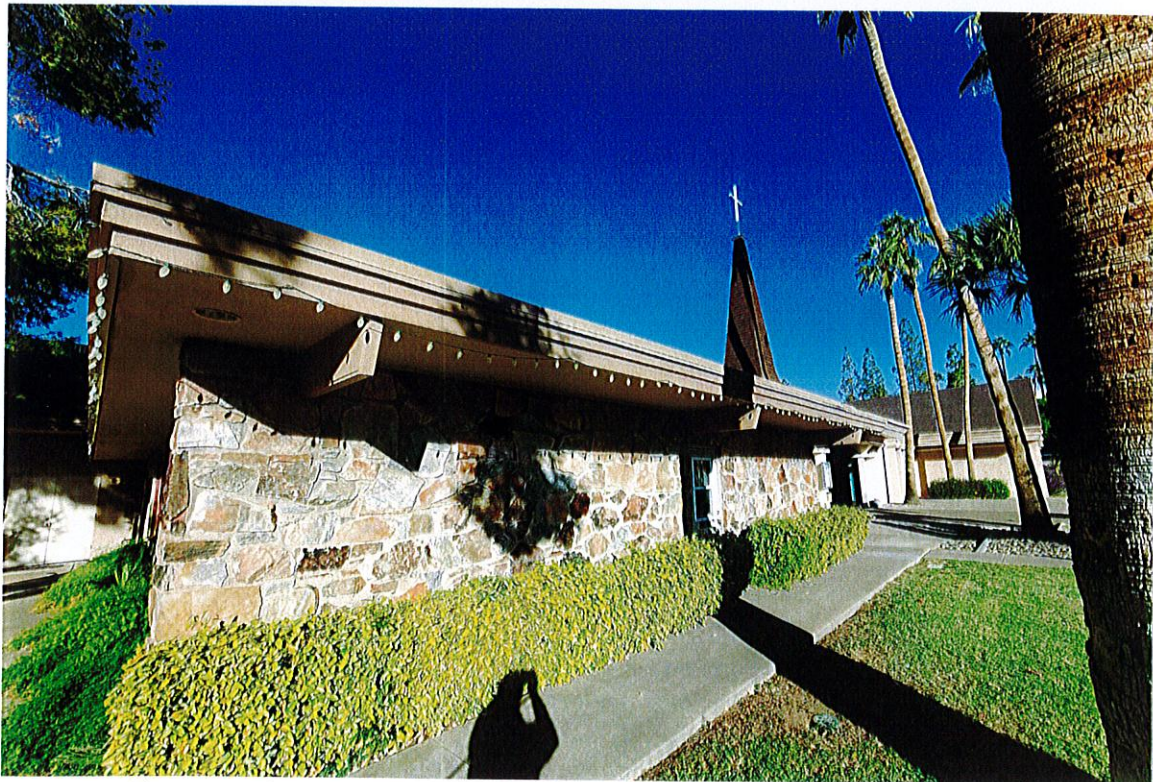
Photo OS12: Close-up of stone veneer on east end of office wing. This was a popular application in the late 1950s. Stone appears to be schist from desert mountains.
