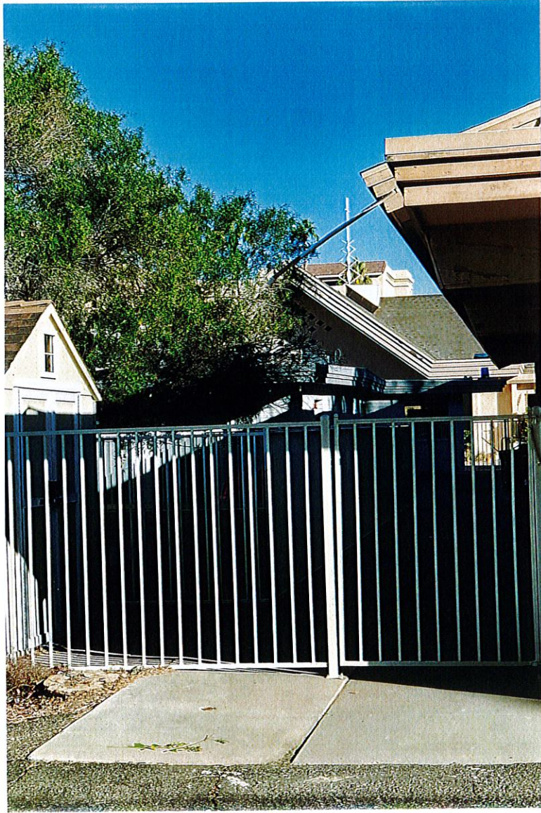
Photo OS6: Southwest corner of original sanctuary looking north to walkway separating education wing and new sanctuary in background.
