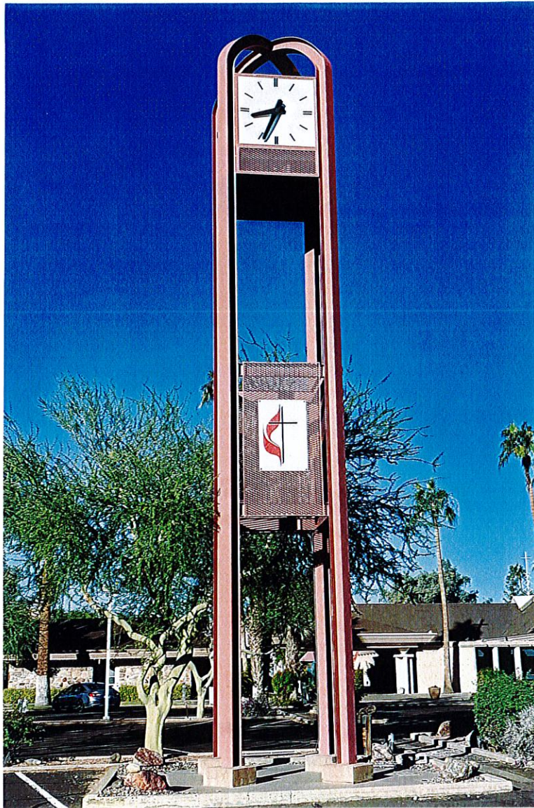
Photo S4: The clock tower in the east side parking area (south of main entry drive), looking west. This is built with steel I-beams.
