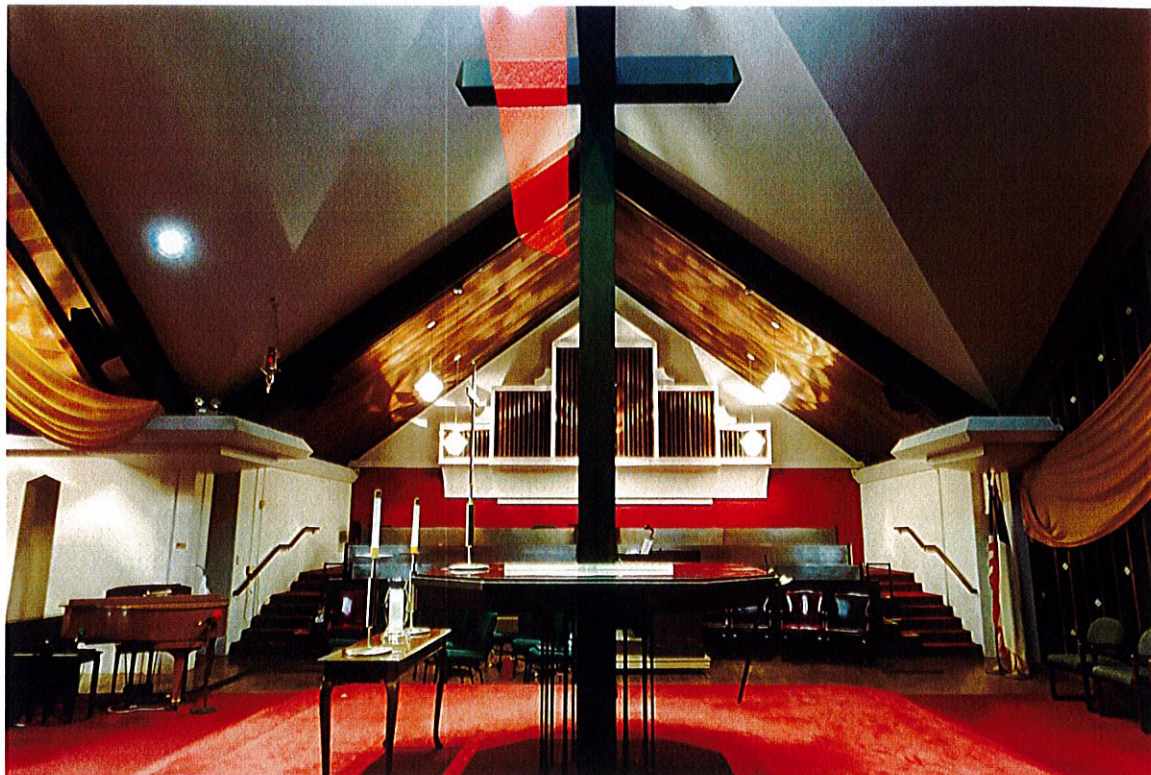
Photo NS26: Looking west toward choir area from the dais. The pipes for the organ have been removed.
