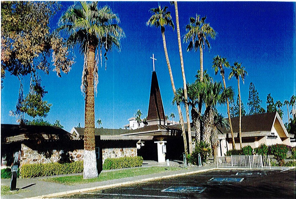
Photo NS6: The entry ramada looking from the southeast.
