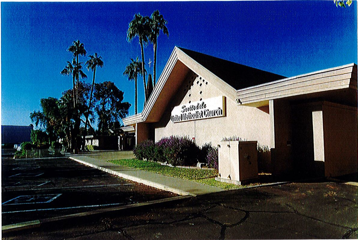
Photo NS1: The northeast corner of the new sanctuary building. The end panel appears to be composed of concrete panels placed over wood frame and then stuccoed.
