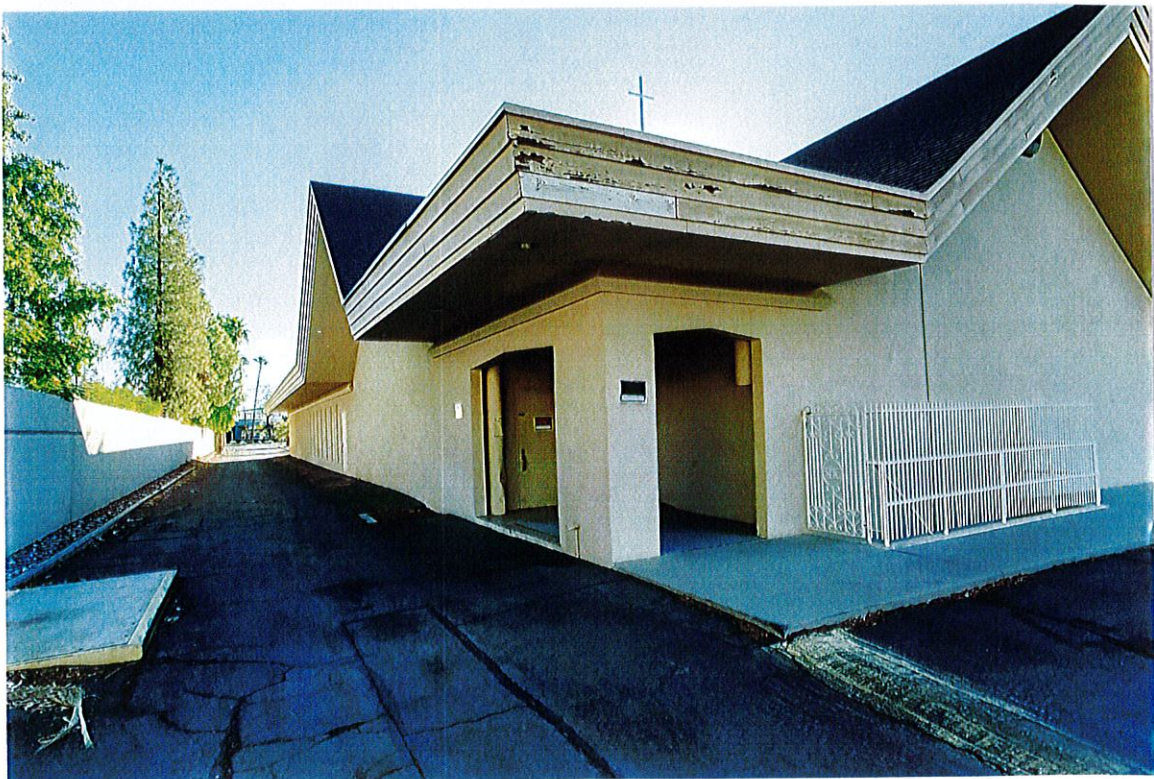
Photo NS9: The northwest corner of the new sanctuary building and the service access.
