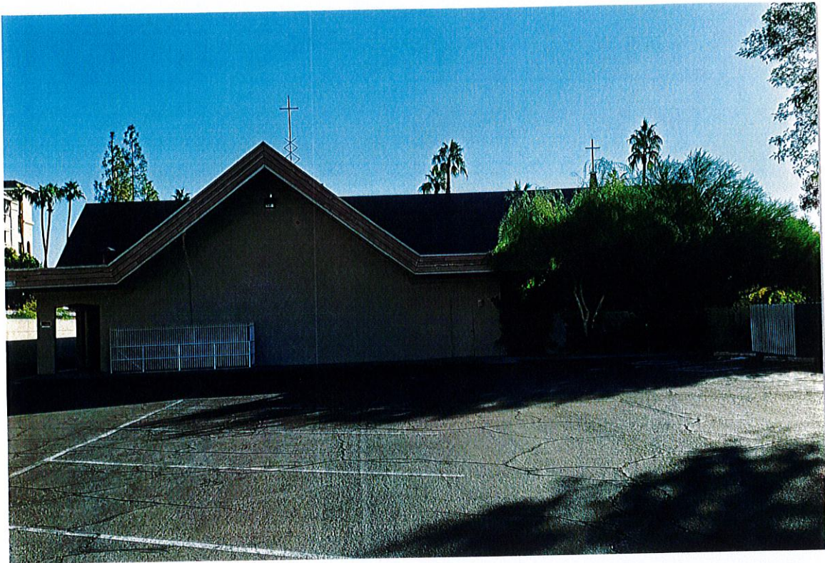
Photo NS8: The west end of the new sanctuary building. The wrought-iron fence encloses access to the lower mechanical spaces.
