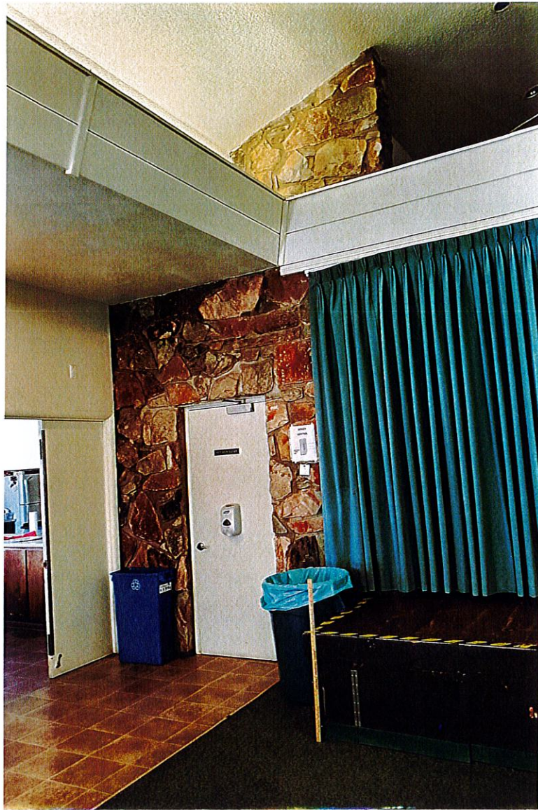
Photo OS18: Close-up of stone veneer that flanks the stage area in the original sanctuary space.
