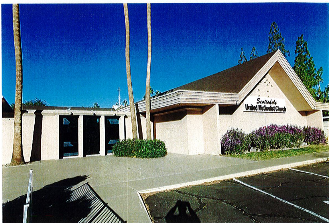
Photo NS4: The southeast corner of the new sanctuary with the foyer on the left.
