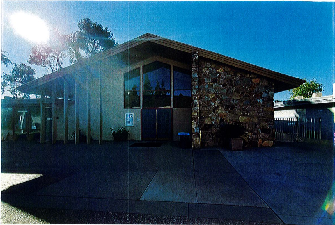
Photo OS13: North (entrance) end of the original sanctuary building. Note the use of stone veneer, vertical wood slat columns and triangular windows (original cross next to entry has been removed).
