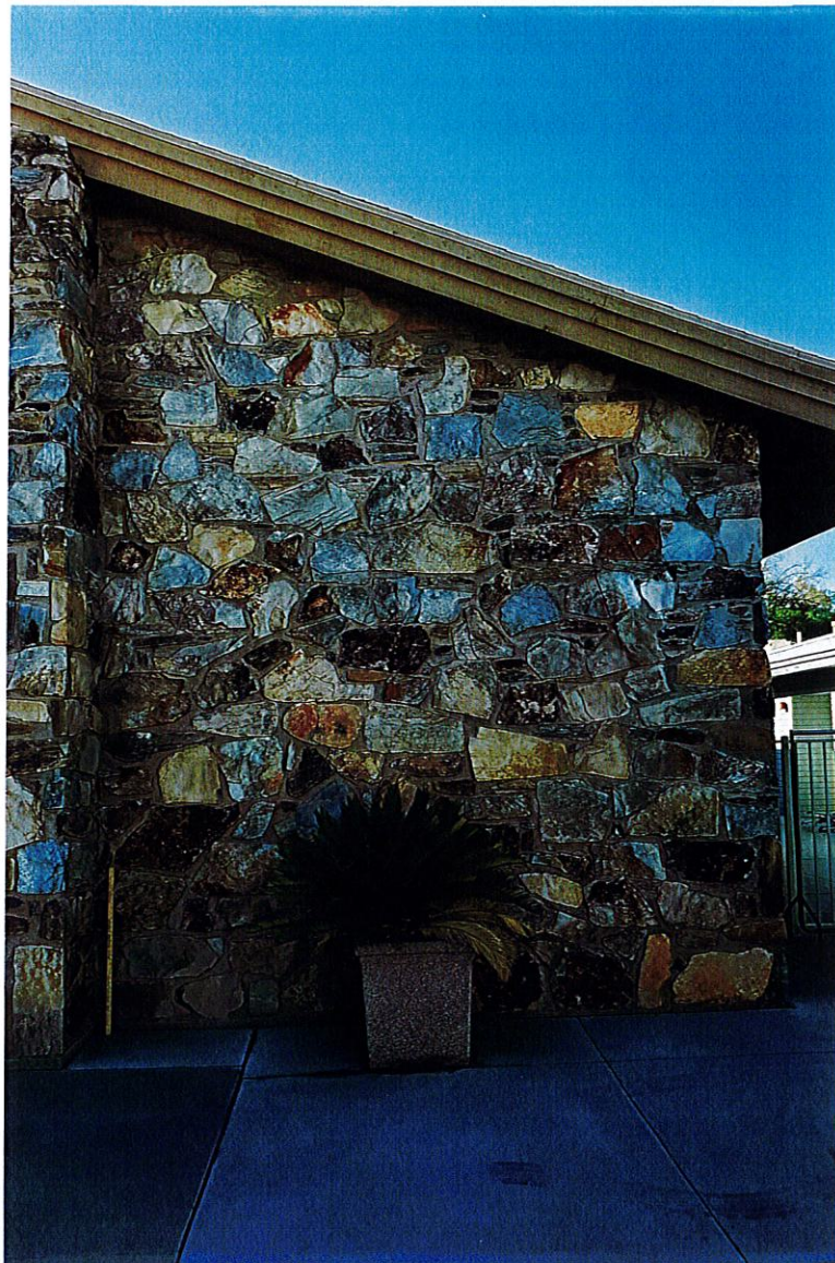
Photos OS14: Close-up of the stone veneer on the north side of the original sanctuary.
