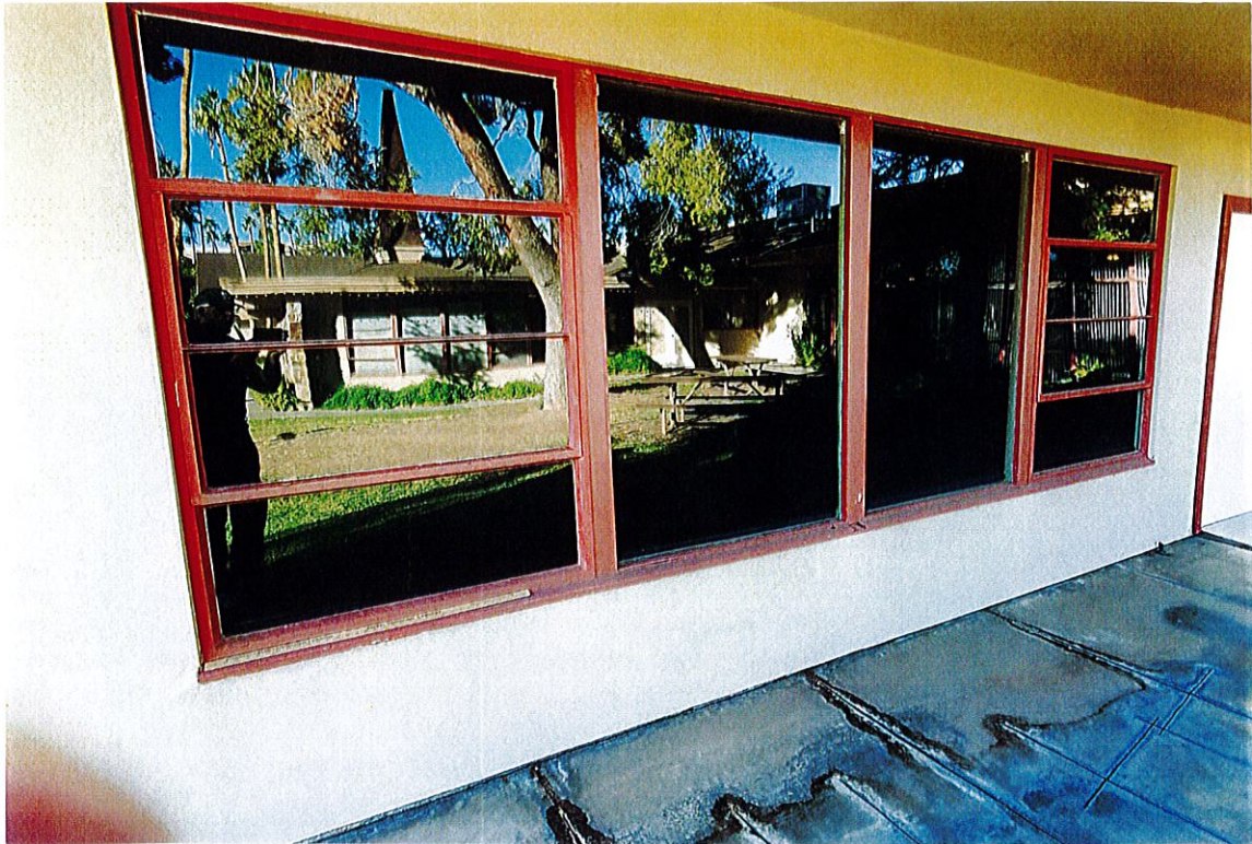
Photo OS7: Steel casement window on north side of office wing. The center sections of left and right panels are operable, which was common to allow ventilation of evaporative coolers.
