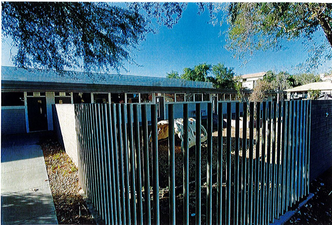
Photo E3: The north side of the new education building as seen from the northeast corner of the play area.
