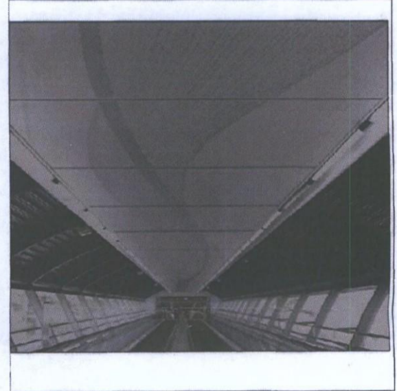
MTL-3 METAL: COMPOSITE ALUMINUM PANEL W/ SCREEN PRINTED PATTERN (SIMILAR TO ABOVE PHOTO)
