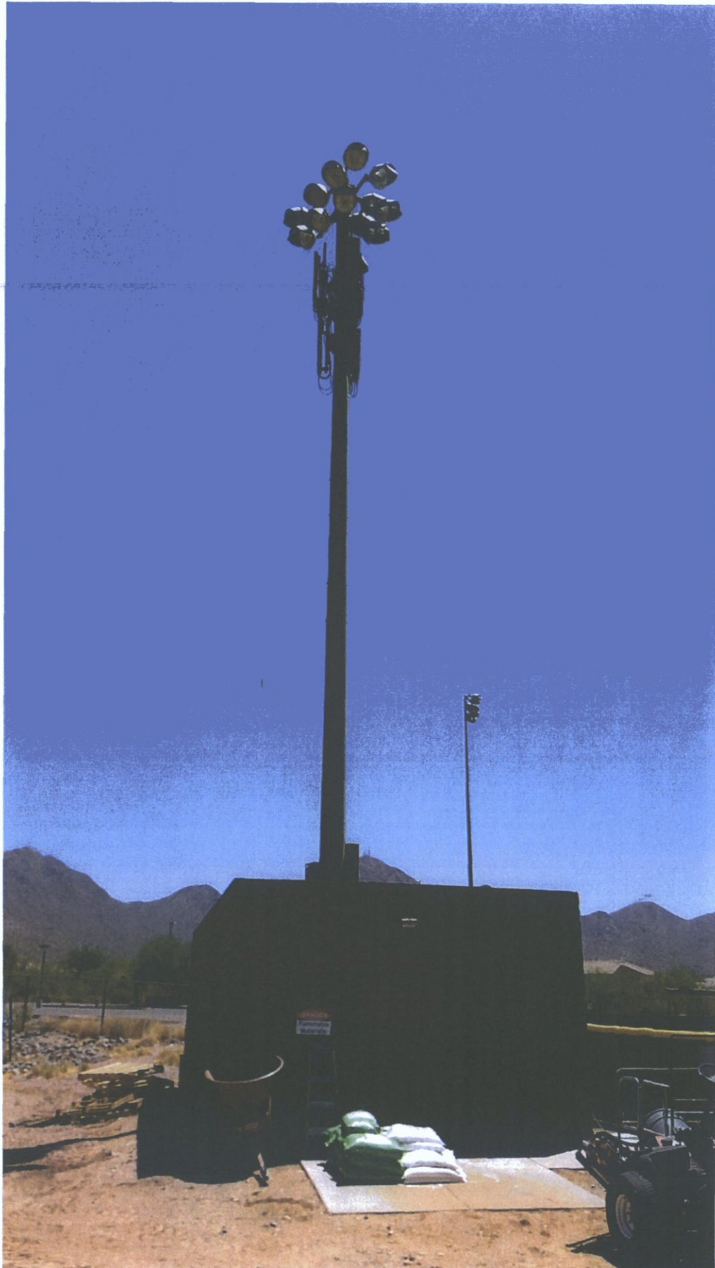
Photo 18 – View of Tower ATTACHMENT #4
