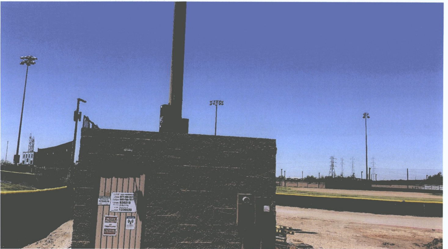
Photo 8 – East Side of Site – Looking West
