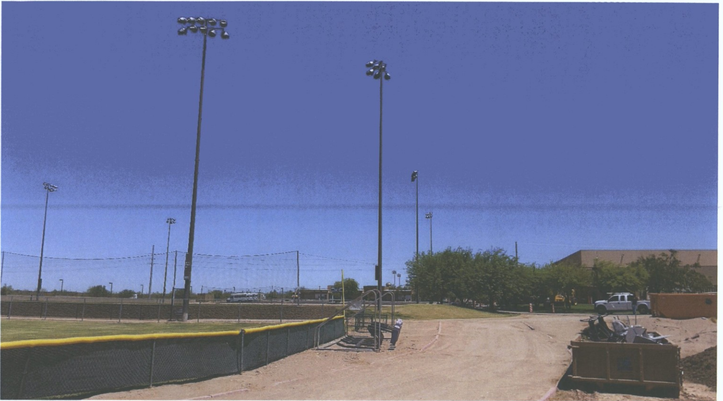
Photo 13 – West Side of Site – Looking North
