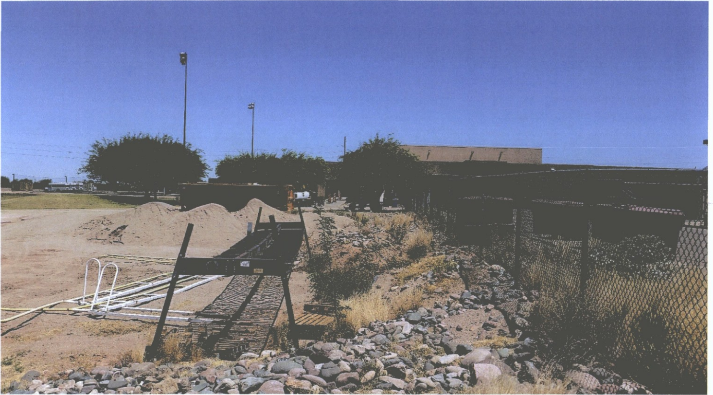
Photo 5 – East Side of Site – Looking North
