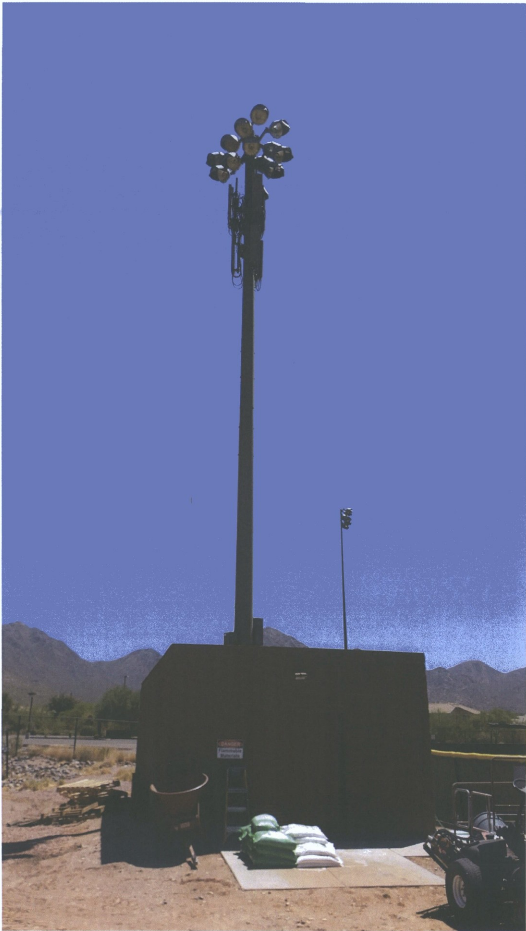
Photo 18 – View of Tower
