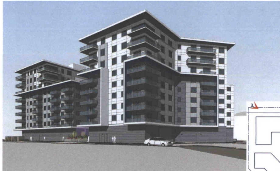
4. VIEW TOWARDS SOUTH TOWER, LOOKING NORTH EAST
