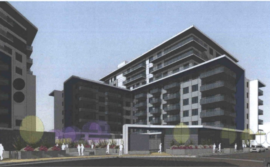
1. VIEW TOWARDS MAIN ENTRANCE LOOKING NORTH EAST
