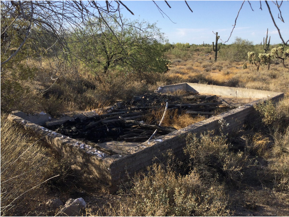
Figure 19e.2. IO #1, historic structure foundation; view is to the south.
