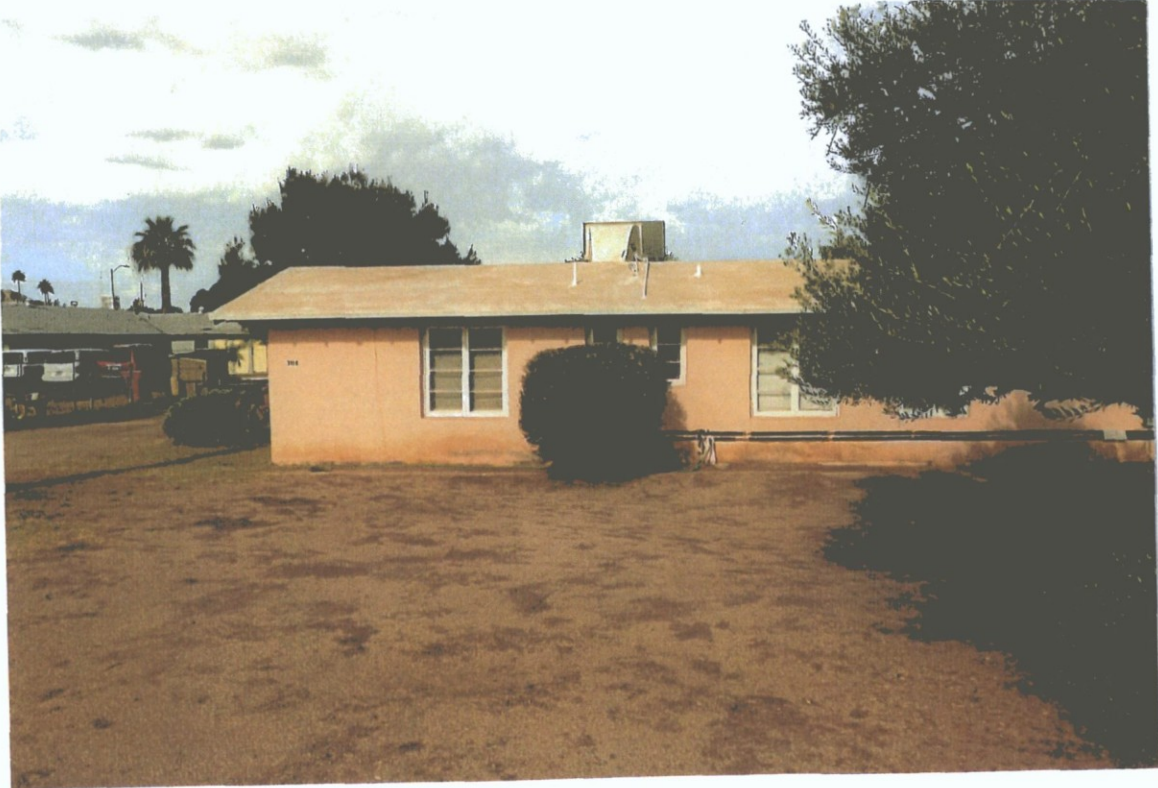
East side looking west
