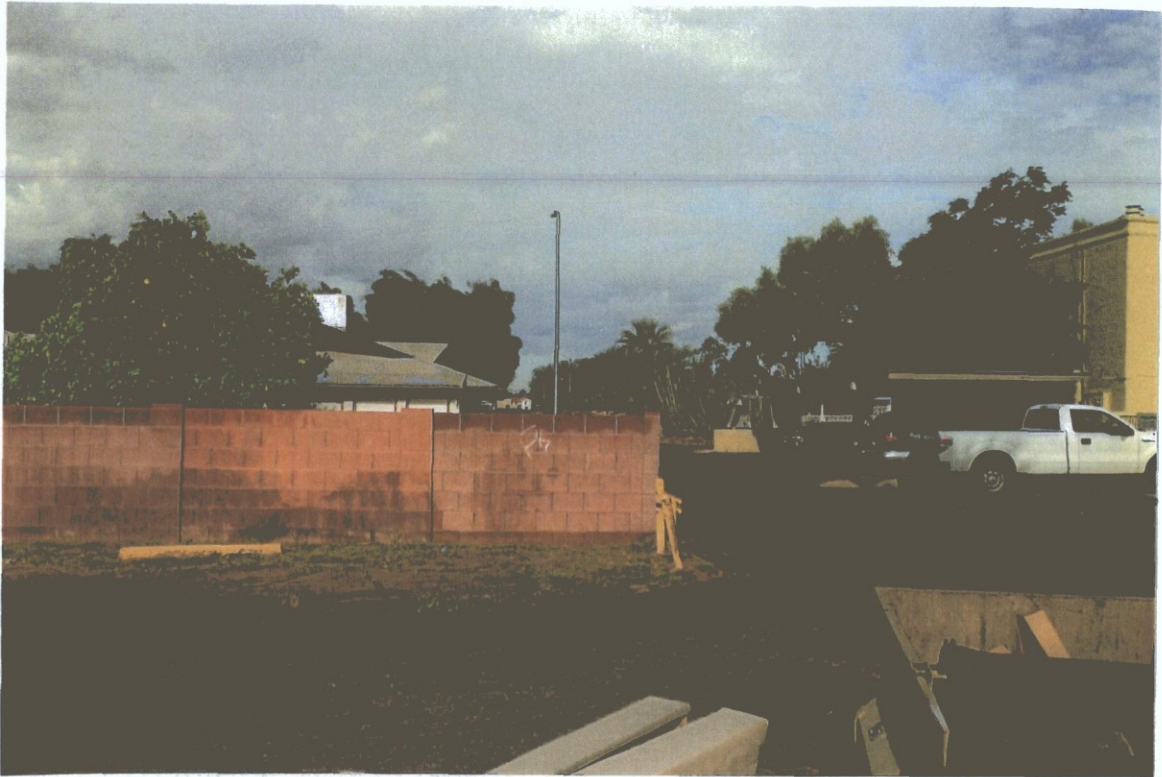
Northwest corner looking west
