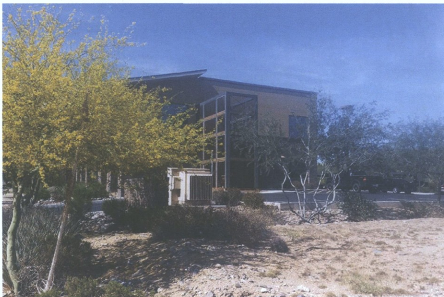
DIGITAL SYSTEMS FROM SITE LOOKING NORTHEAST
