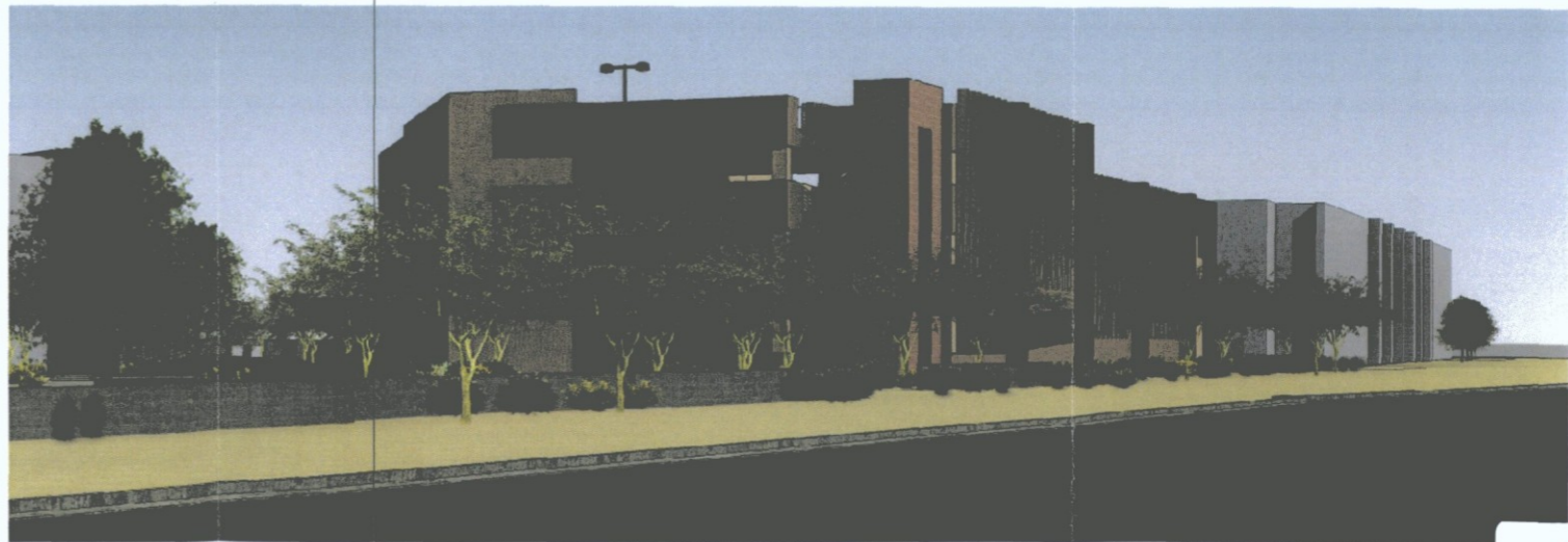
3 View From Intersection
