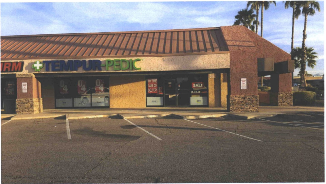
#1 – North side of site looking north
