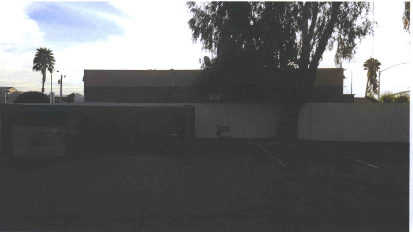
#14 – West side of site looking east
