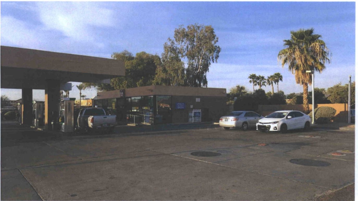
#4 – North side of site looking southwest
