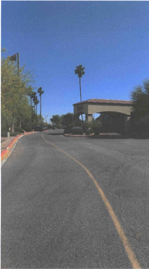
Photo #9 Northeast Corner of site looking West
