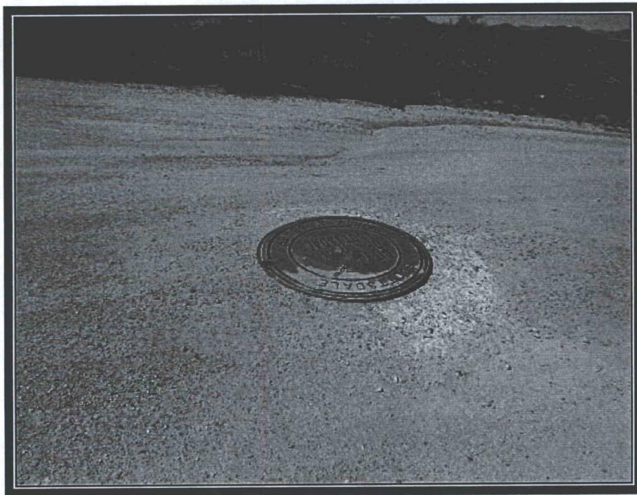
Manhole in 128 th Street
