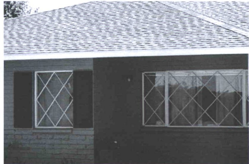
Some steel casement windows in Village Grove have the decorative diamond pane pattern. Shutters also flank some windows on the front façade.
