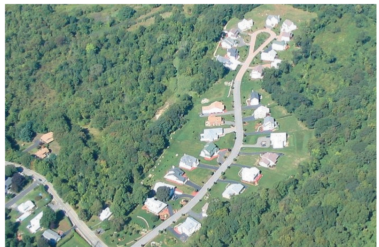
By eliminating detention pond, the subdivision layout conserves trees while 15,000 sf (1500 m 2 ) PICP in the cul-de-sac returns rainfall to the water table in Glen Brook Green subdivision in Waterford, CT.
