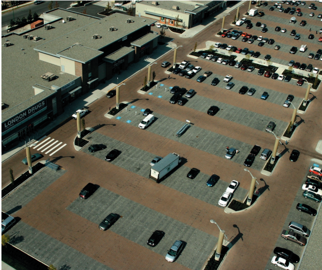
350,000 sf (3.2 ha) of PICP at a Burnaby, BC shopping center infiltrates runoff from roofs.
