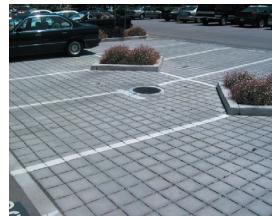
Pavers are delivered ready to place, joints filled, compacted and then are ready for traffic.
