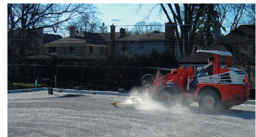
Mechanical sweeping of fine aggregate into paver joints
