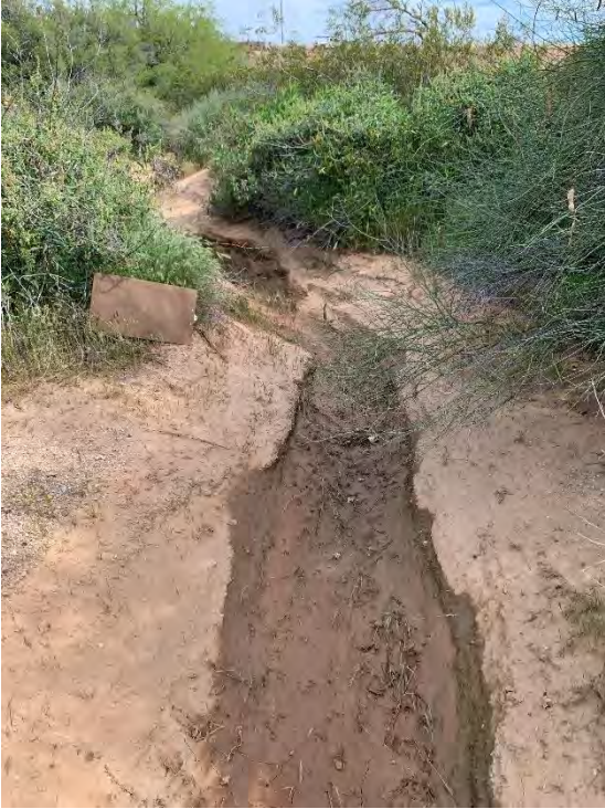
Upstream view facing northeast
