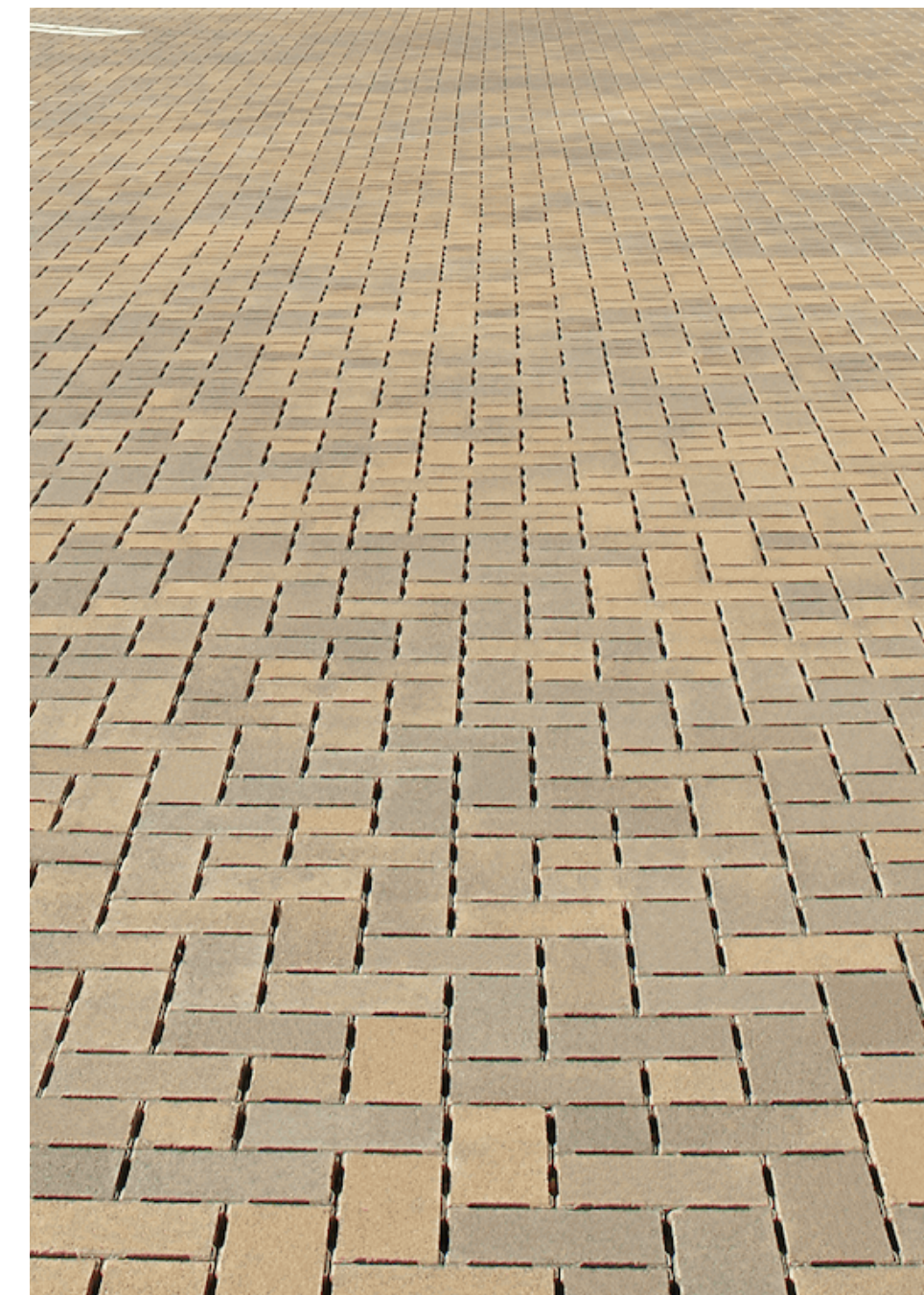
PRECAST CONCRETE PAVERS AT PARKING
