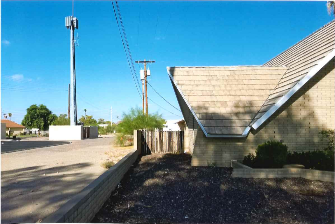
17. Southeast corner looking West
