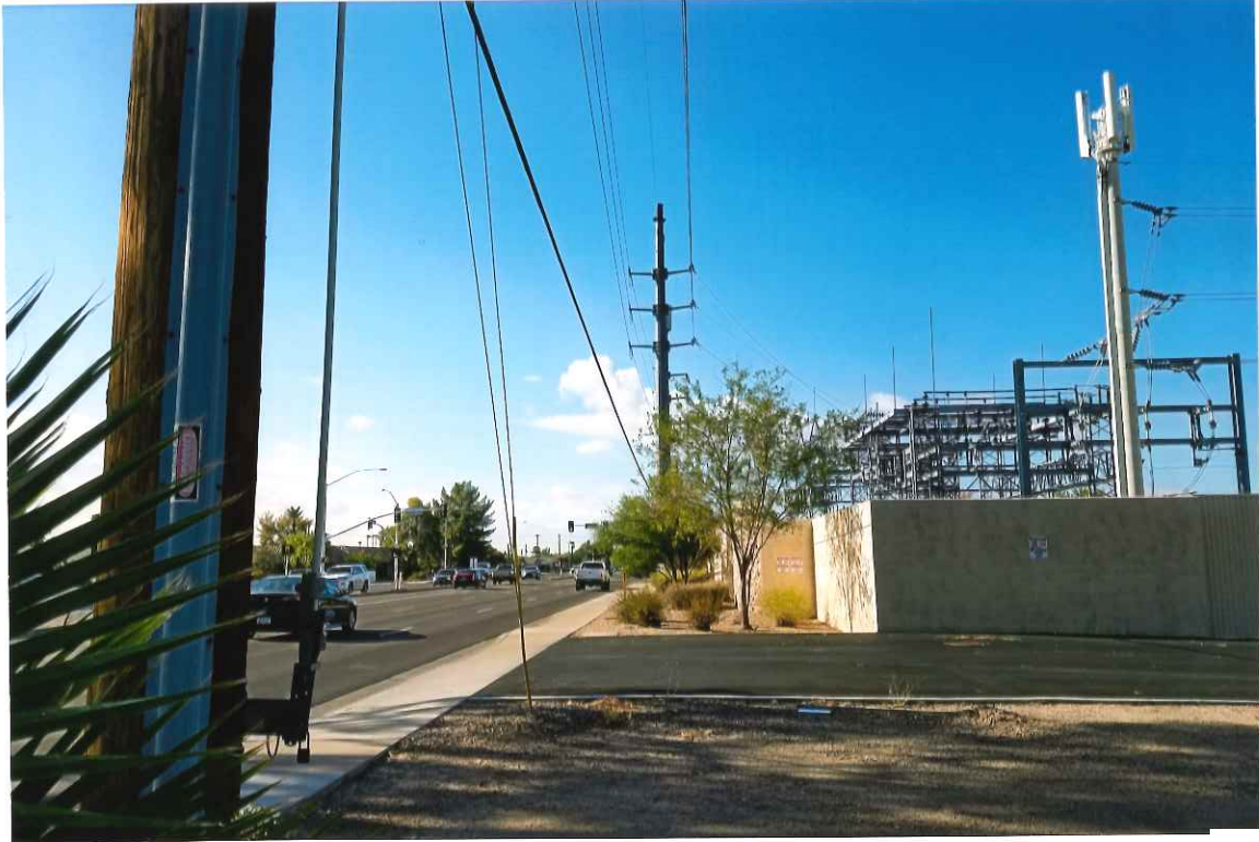
18. Southeast corner looking South
