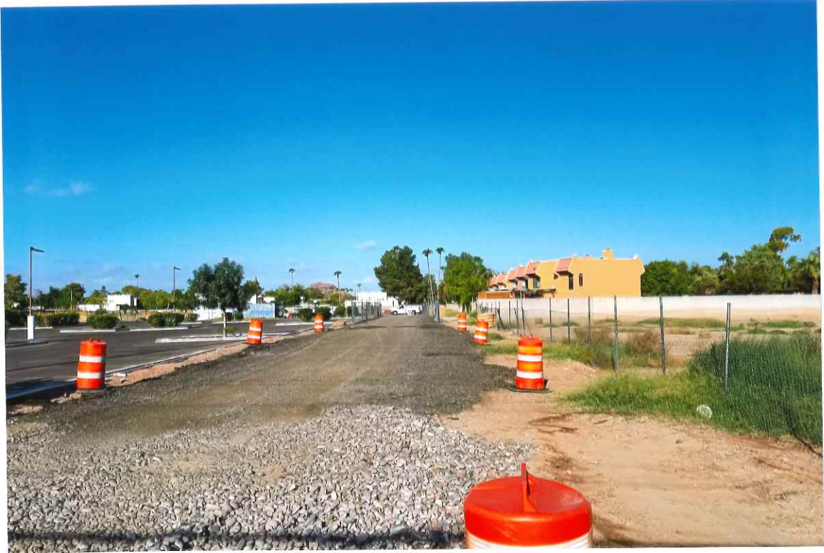
13. Northeast corner looking West
