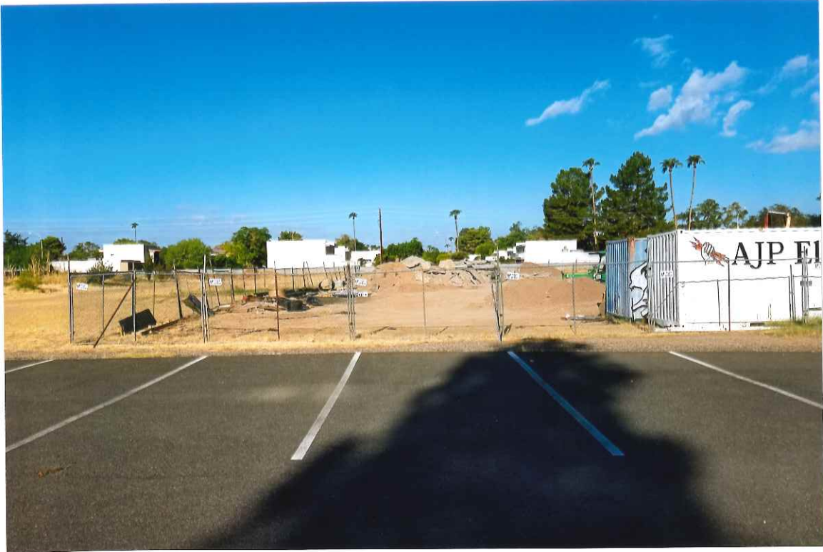
9. Center of Site looking West
