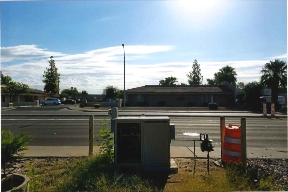
15. Northeast corner looking East
