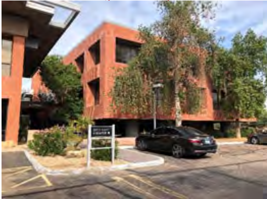
Looking Northeast At Subject
