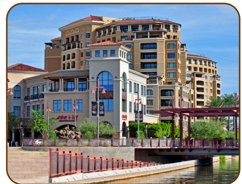
Type 3 development is the highest scale of development permitted and often includes public open and event spaces at the pedestrian level.
