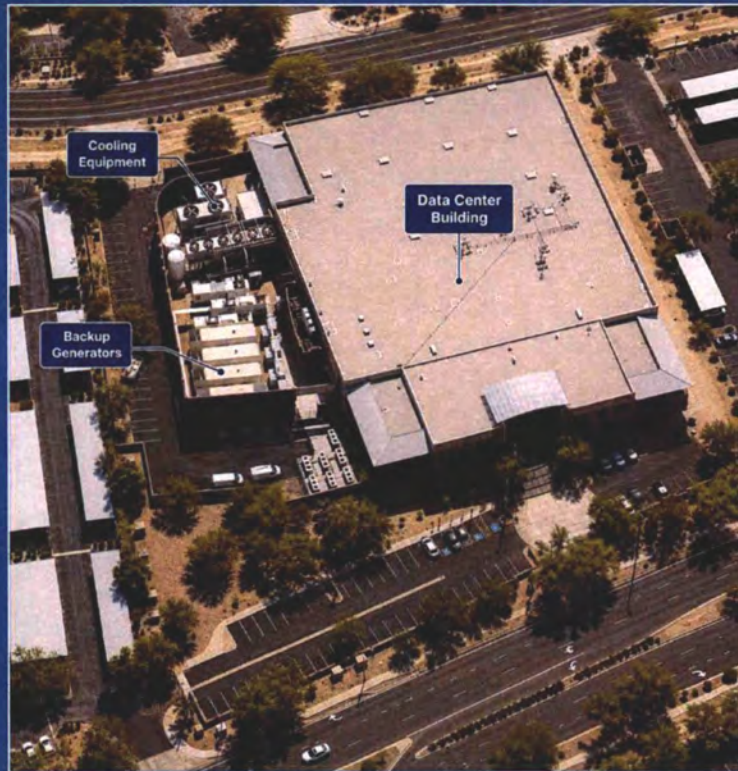
8521 E. Princess (Perimeter Center) +/- 4.5 acres | ~74,000 SF | 5.8+ MW | ~55,000 GPD
