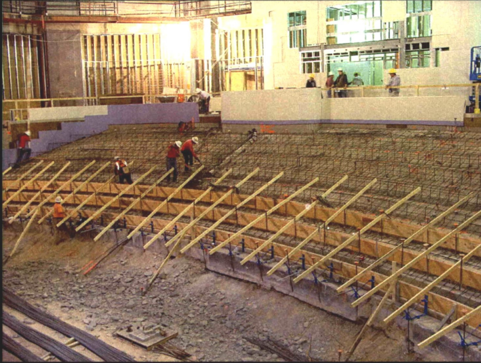
Main Theater Renovations
