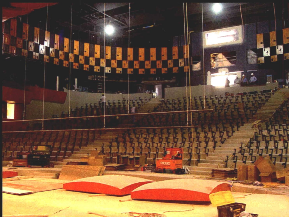
Main Theater Renovations
