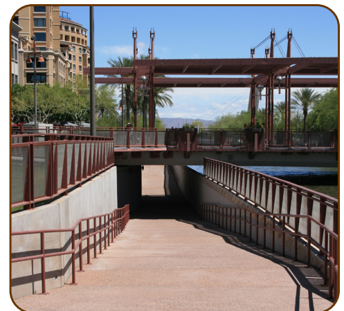
The Marshall Way Bridge underpasses provide increased connectivity along the canal in Old Town.
