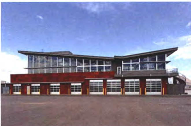
Airport Operations Center Looking North
