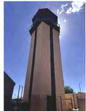
SDL Control Tower
