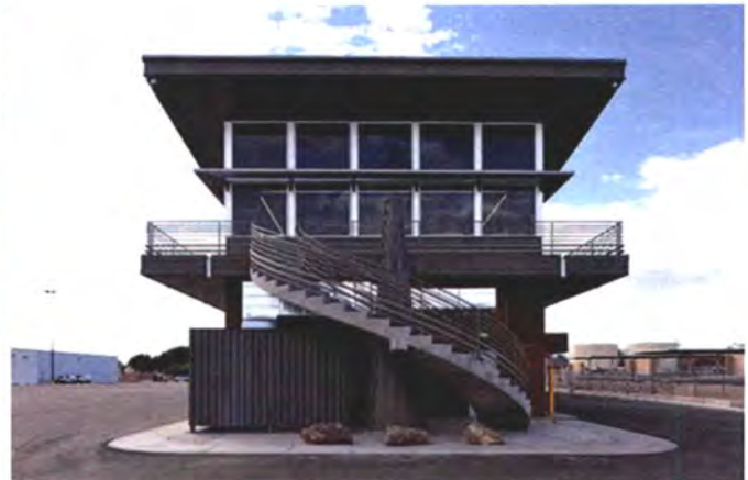
Airport Operations Center Looking West
