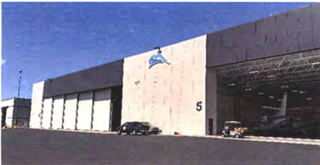
Atlantic Conventional Hangars
