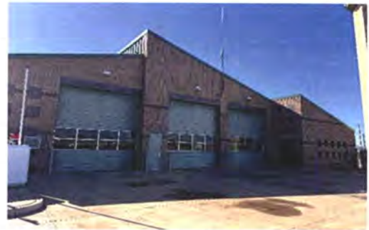
Fire Station 609 at SDL – Airside View
