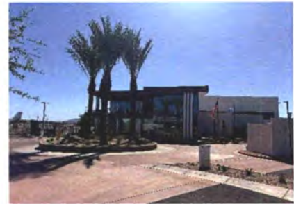
NetJets Office/Hangar Complex
