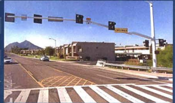
Chaparral Rd and Canal Crossing
