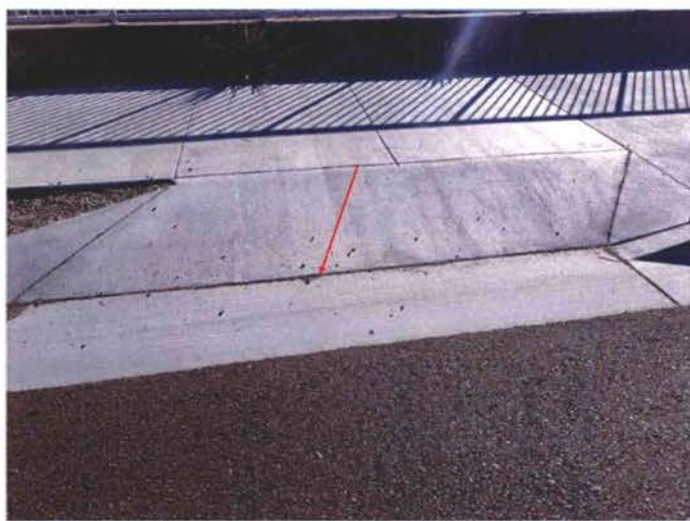
Figure 10: Perpendicular/Directional Curb Ramp with 17.5% Running Slope
