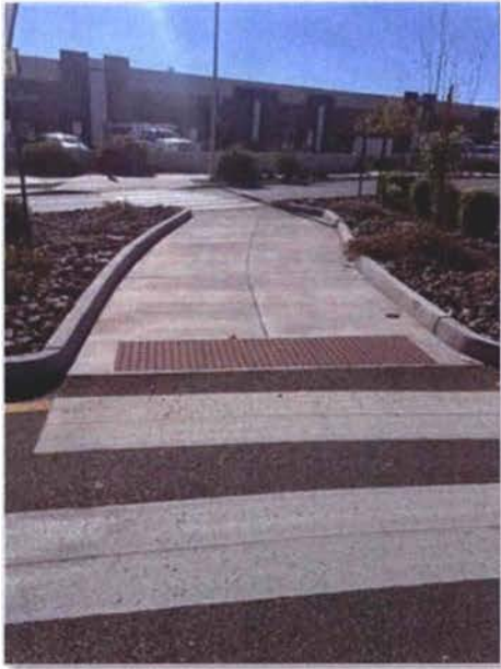
Figure 15: Fully Compliant Median Refuge Island
