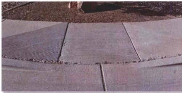
Figure 13: Diagonal Curb Ramp with Textured DWS
