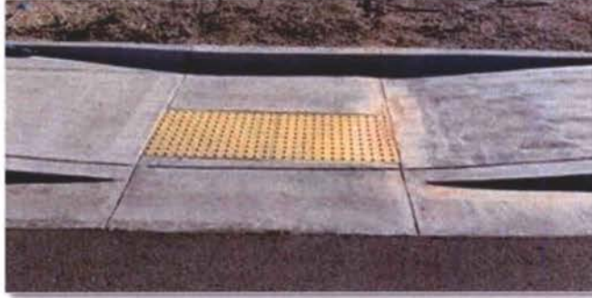
Figure 12: Diagonal Curb Ramp with Domed DWS
