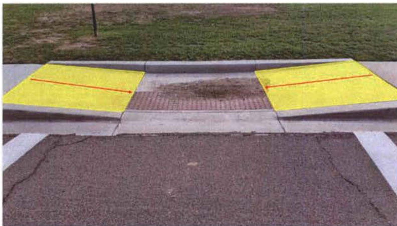
Figure 9: Running Slope Diagram on a Curb Ramp
