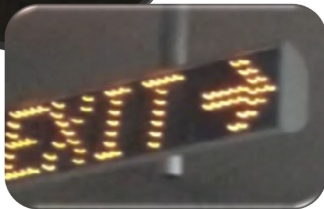
Signs have built in light meters and auto adjust.
