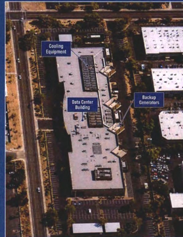
7499 E. Paradise Lane (Greater Airpark) +/- 7.9 acres | ~99,000 SF | 11+ MW | ~3,500 GPD
