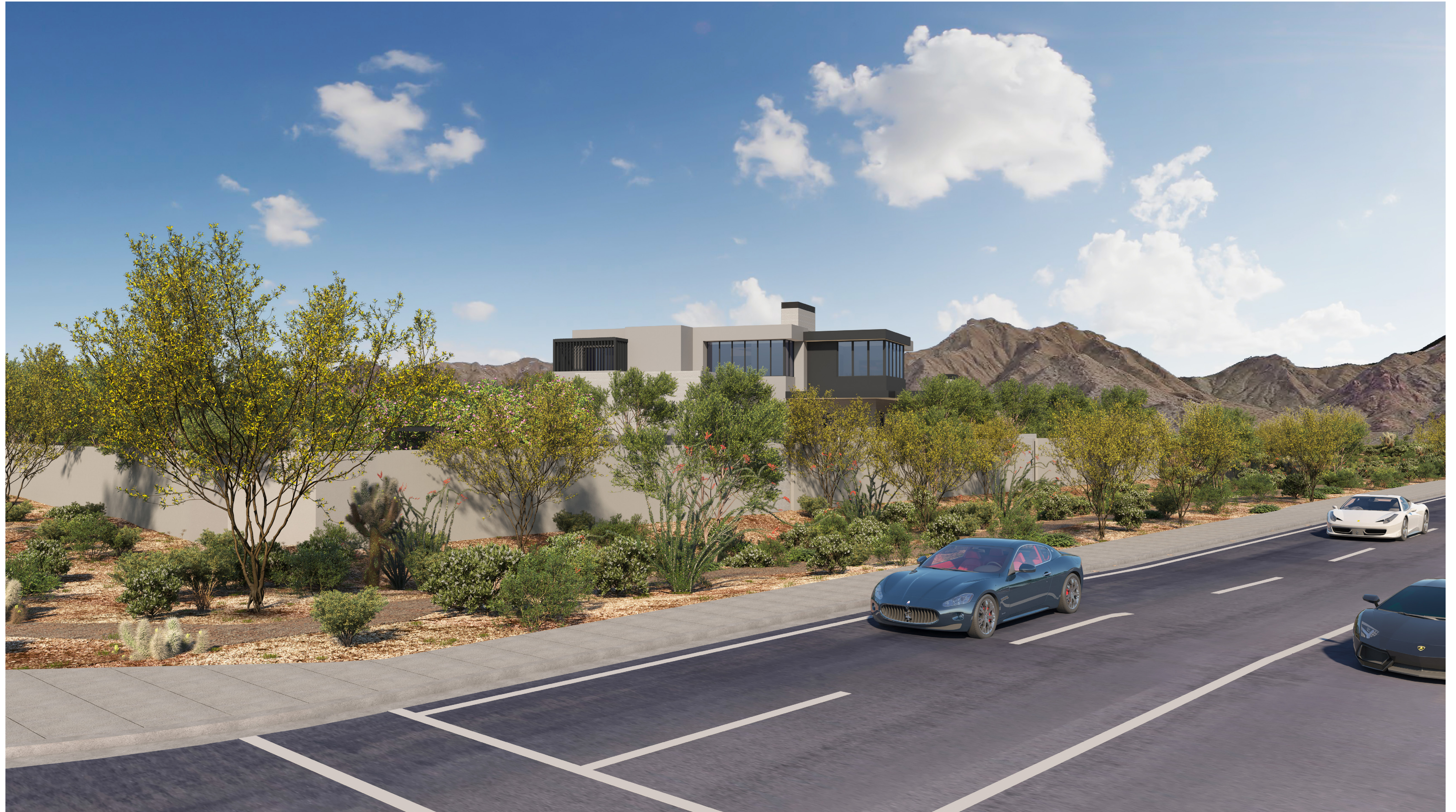
STREET VIEW OF CLUBHOUSE FROM CORNER OF 94TH STREET AND BELL ROAD
