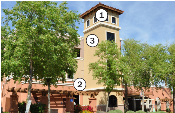
5th Avenue public parking garage.
