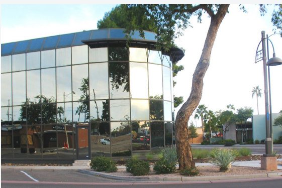
DISCOURAGED - The mirrored glass clad building lacks transparency, causes glare, and does not project a desert southwest character or sense of place.
