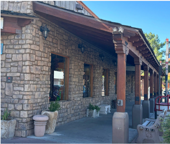
The clear glass windows of this retailer are deeply recessed into the stone wall, providing a sense of the wall massing.
