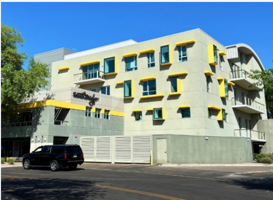
ALTERNATIVE OPTION - ALTHOUGH FACING A PUBLIC STREET THE service AREA occurs within a SCREENED courtyard-screened from the street.
