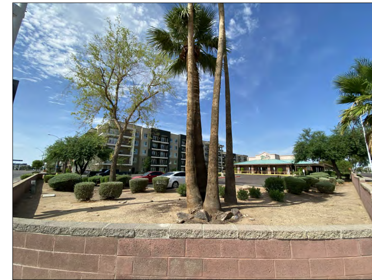
VIEW 8 From Intersection of E. Osborn Rd. and N. Scottsdale Rd. Looking SW
