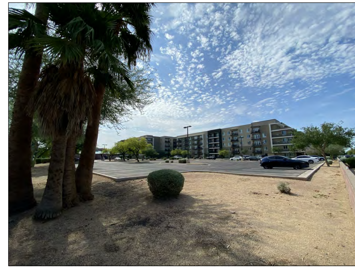
VIEW 2 From East Osborn Rd. Looking SE
