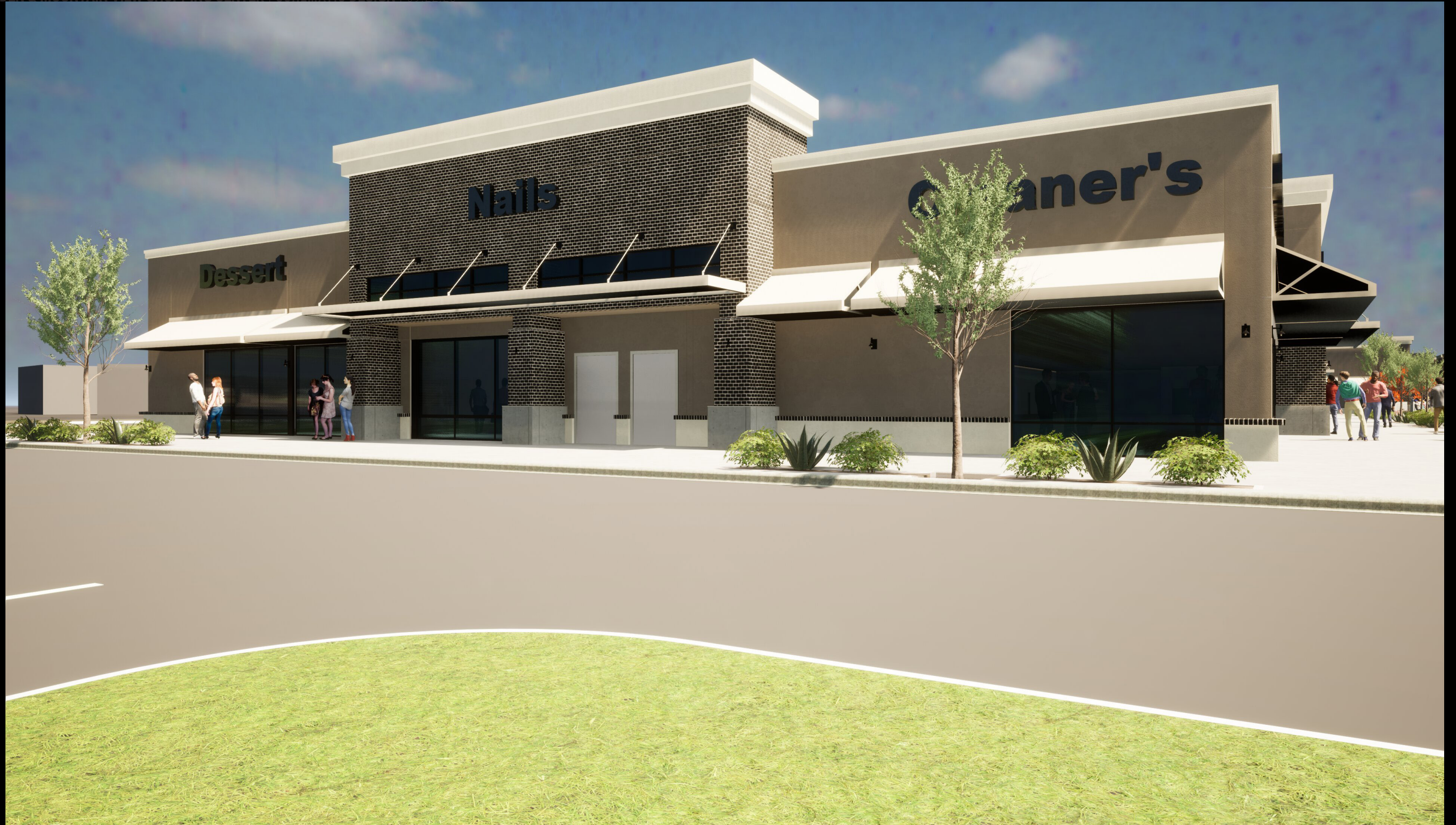
VIEW 13 BUILDING C
