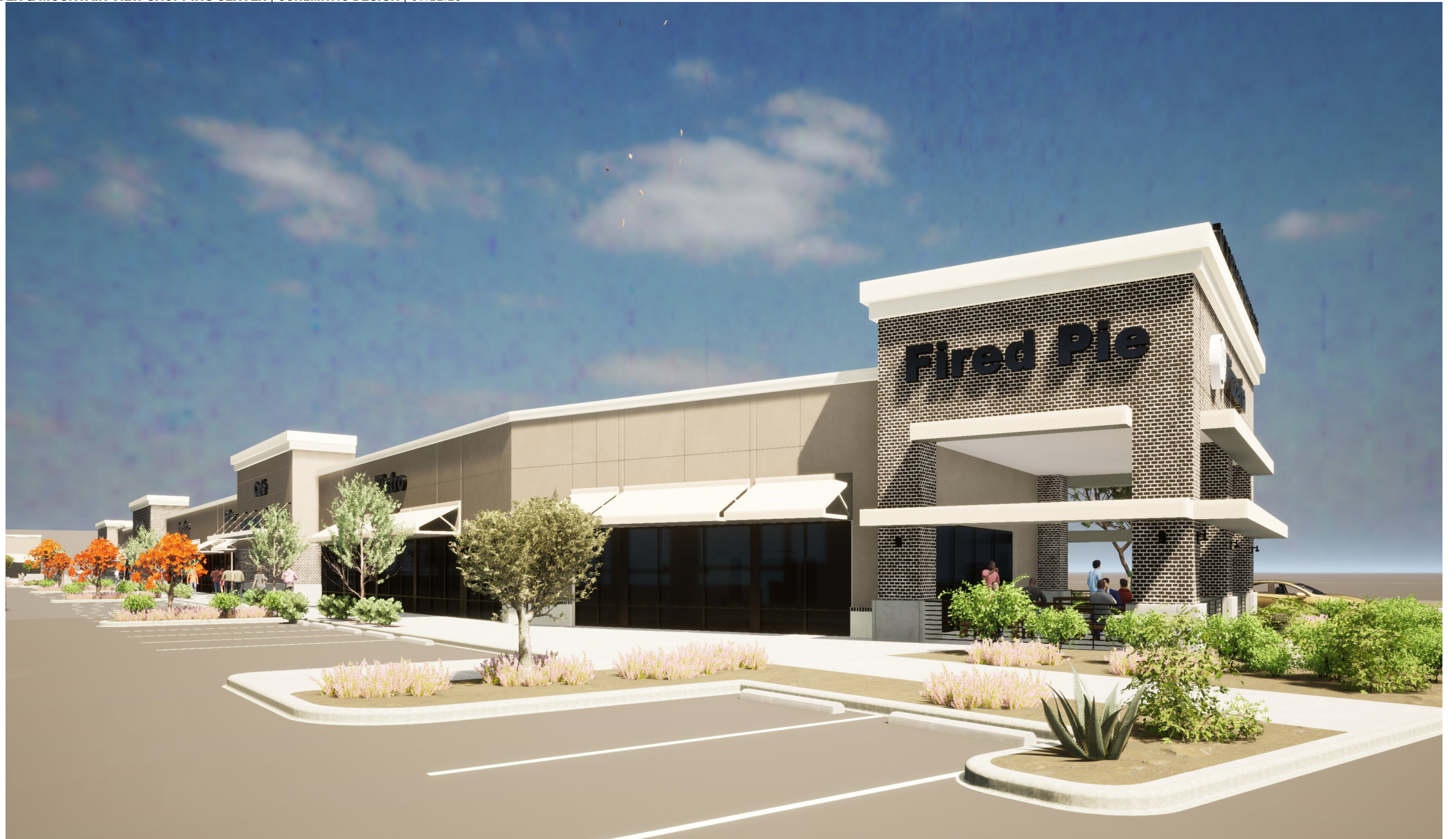
VIEW 1 BUILDING A
