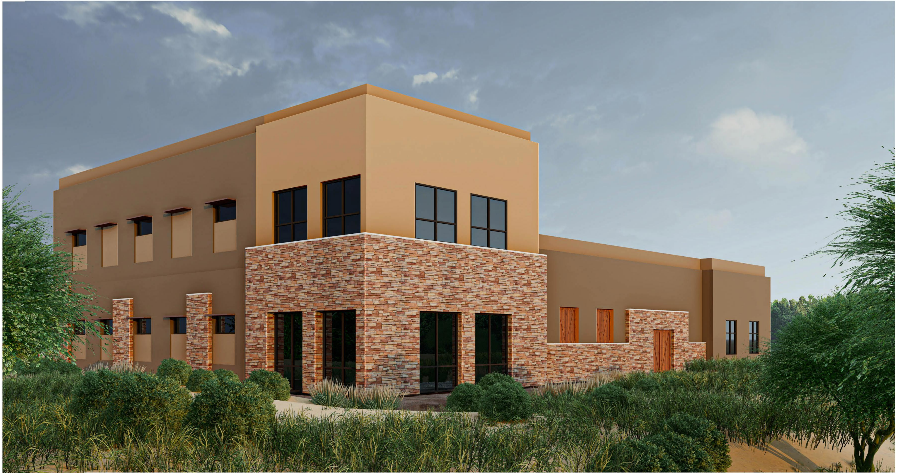
BUILDING FRONTAGE - SE CORNER VIEW
