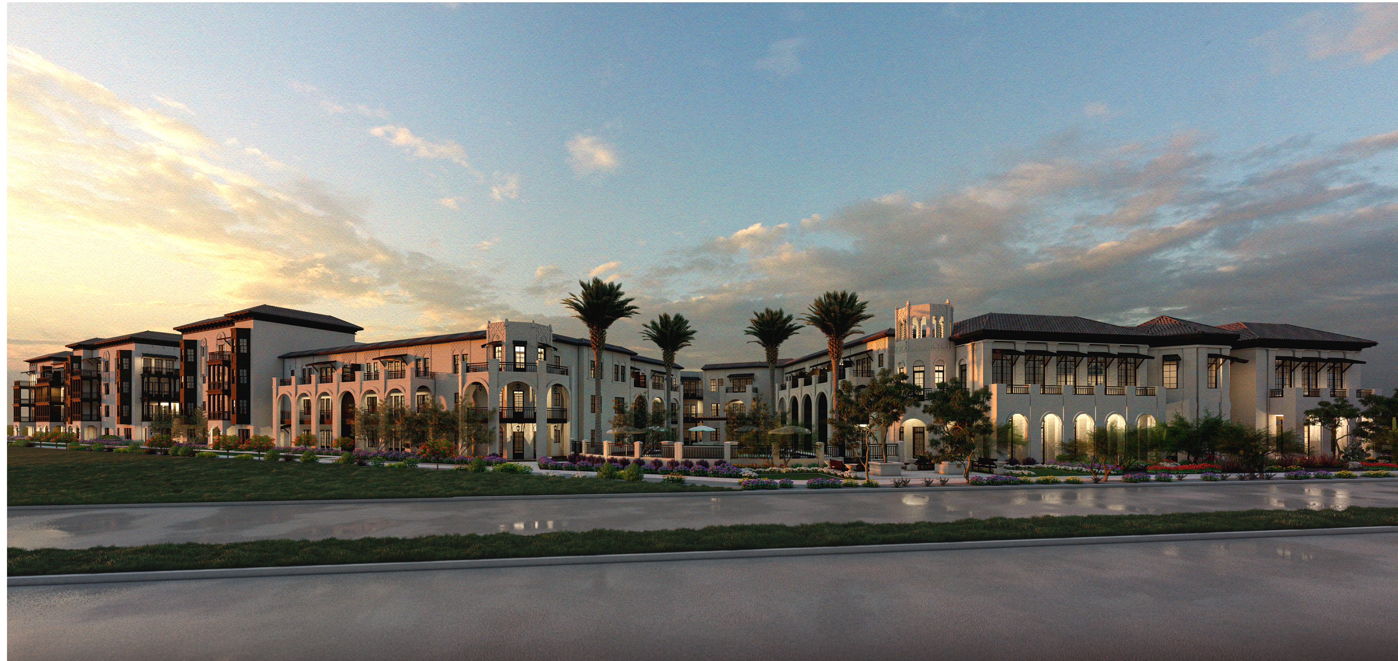
1. VIEW FROM NORTH EAST
