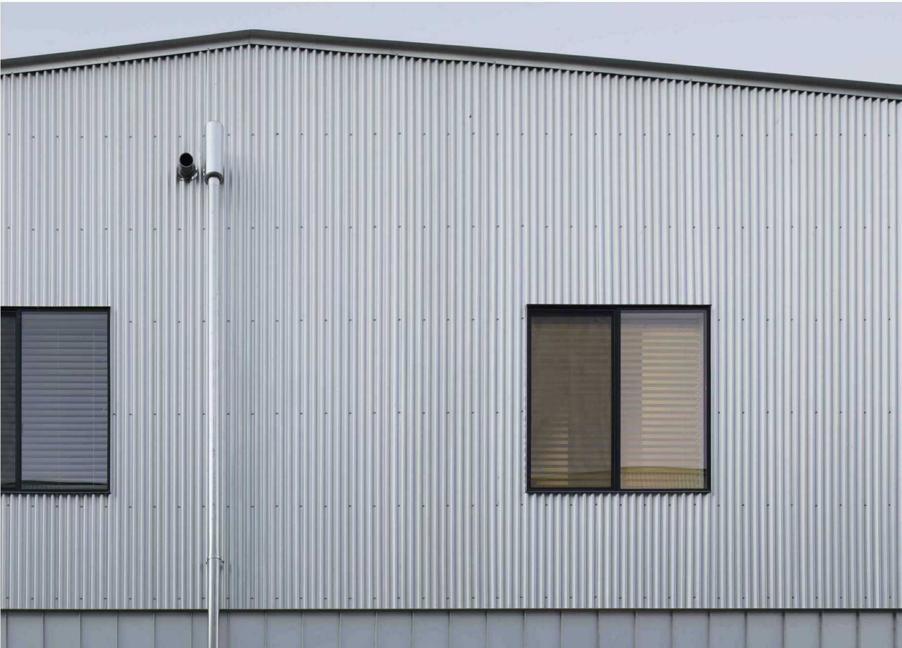
[MTL-2] 22GA 7/8" CORRUGATED METAL WALL CLADDING W/ GALVALUME FINISH
