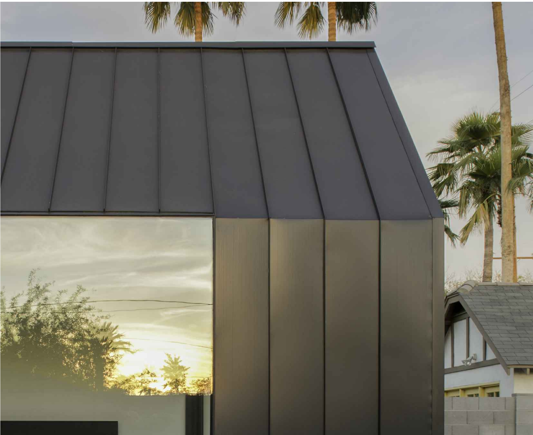
[MTL-1] STANDING SEAM METAL ROOFING W/ KYNAR 500 FINISH
