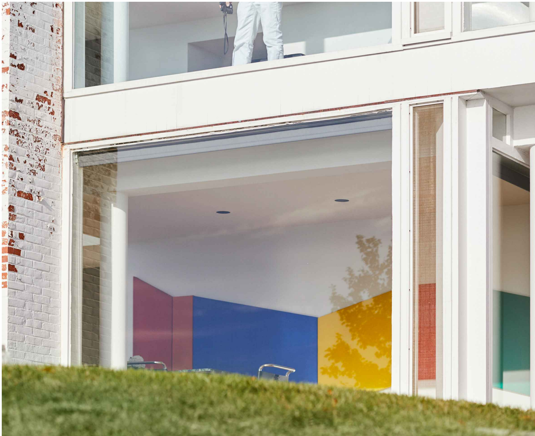
[WIN-1] PTD WHITE THERMALLY BROKEN ALUMINUM WINDOW/DOOR FRAME W/ 1" INSULATED GLAZING WITH LOW-E COATING
