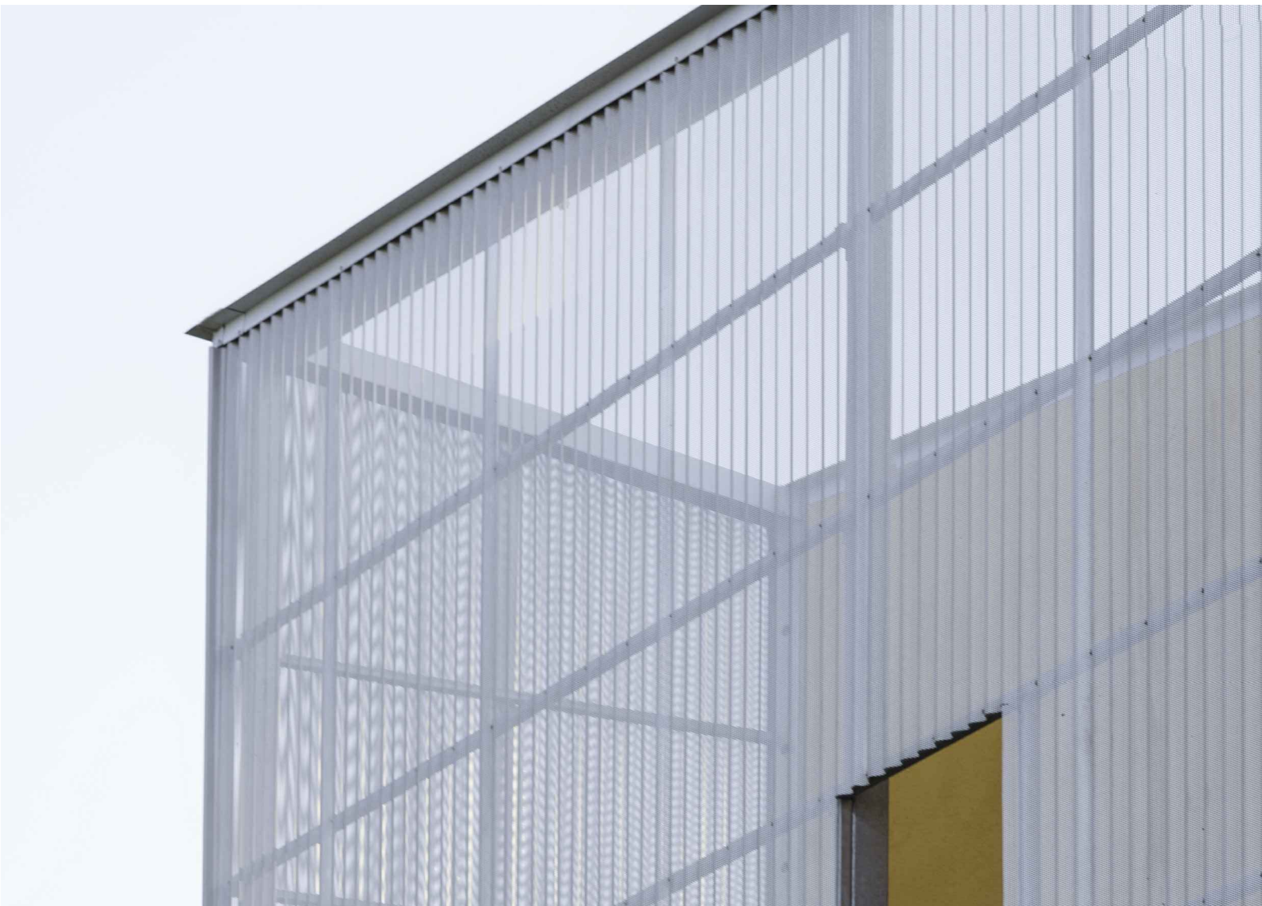
[MTL-3] PERFORATED 22GA 7/8" CORRUGATED METAL WALL CLADDING W/ GALVALUME FINISH
