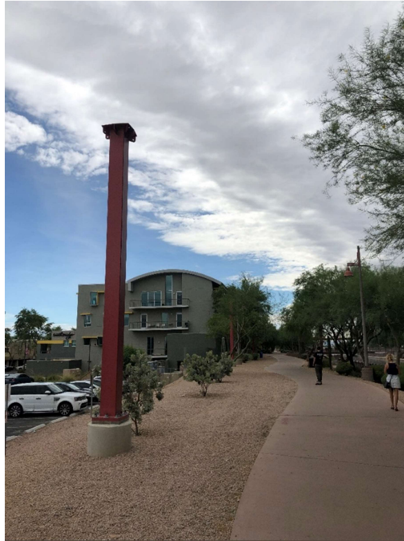
Photo 1 – Existing HSS Steel Tube (Molecules Support Structure)
