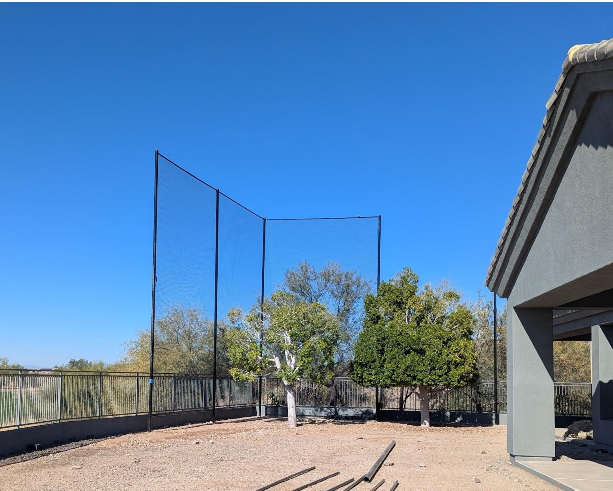
Initial installation – 30 feet
