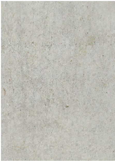
CONC-1 DESCRIPTION: SEALED CONCRETE LOCATION: TILT CONCRETE WALL PANELS COLOR: NATURAL GREY TEXTURE: SMOOTH
