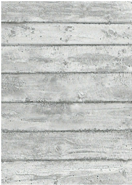
CONC-2 DESCRIPTION: BOARD FORMED CONCRETE LOCATION: TILT CONCRETE WALL PANELS COLOR: STANDARD GREY TEXTURE: BOARD FORM
