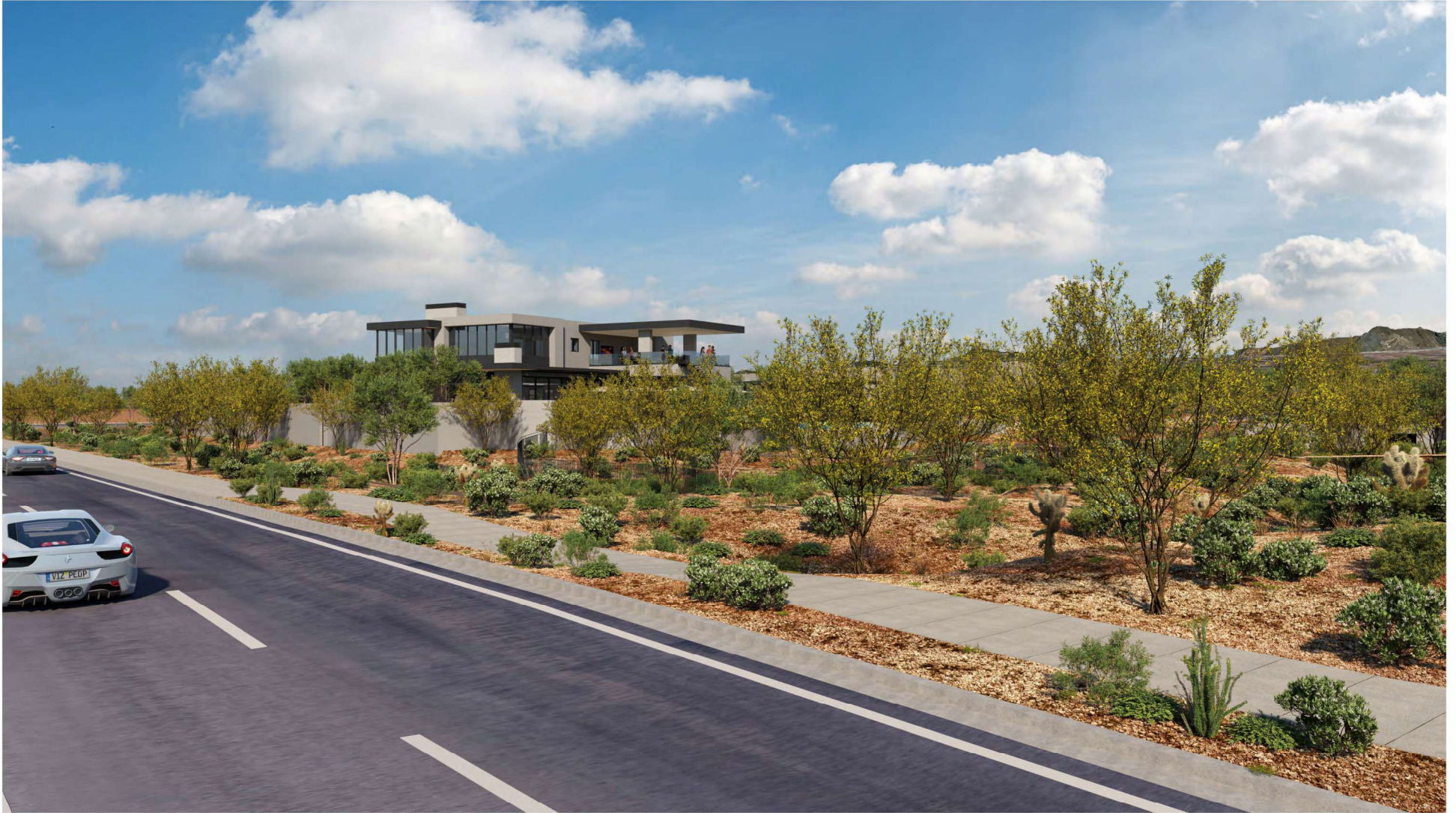
STREET VIEW OF CLUBHOUSE FROM BELL ROAD LOOKING WEST
