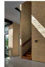
17 BOARD FORMED CONCRETE
