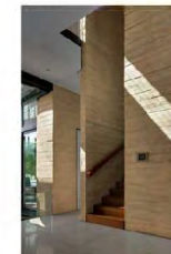
Ⓓ BOARD FORMED CONCRETE
