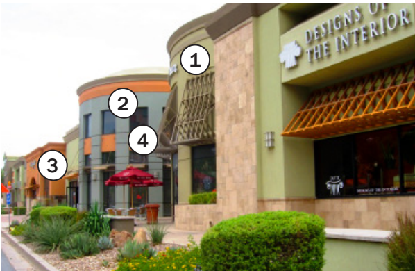
Retail development, northeast corner of Scottsdale and Camelback Roads.
