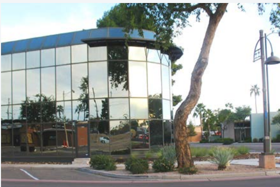
DISCOURAGED - The mirrored glass clad building lacks transparency, causes glare, and does not project a desert southwest character or sense of place.
