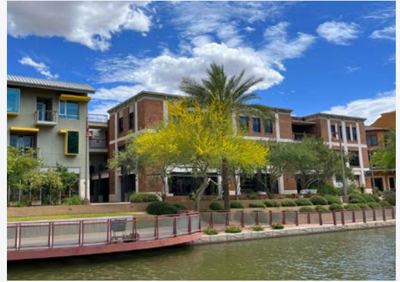
Similar floor-to-floor heights and the alignment of architectural features help define the visual continuity of an area.
