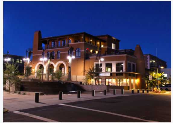
ENCOURAGED - Lighting from the adjoining plaza strategically highlights the architectural features of the building.
