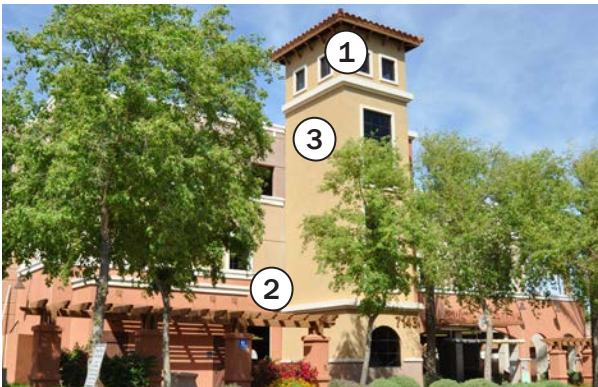
5th Avenue public parking garage.
