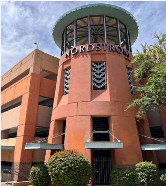
The corner of this parking garage is articulated as a stair tower giving the structure the appearance of a building.
