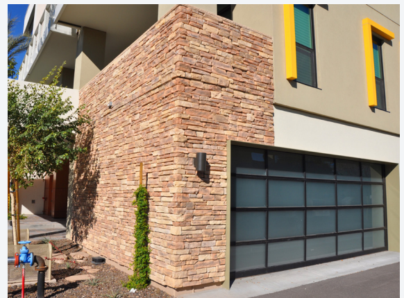
DISCOURAGED - Stacked stone abruptly transitions to smooth stucco, with no horizontal change in wall plane, highlighting the simulated nature of the material.
