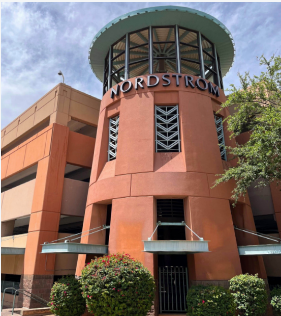
The corner of this parking garage is articulated as a stair tower giving the structure the appearance of a building.
