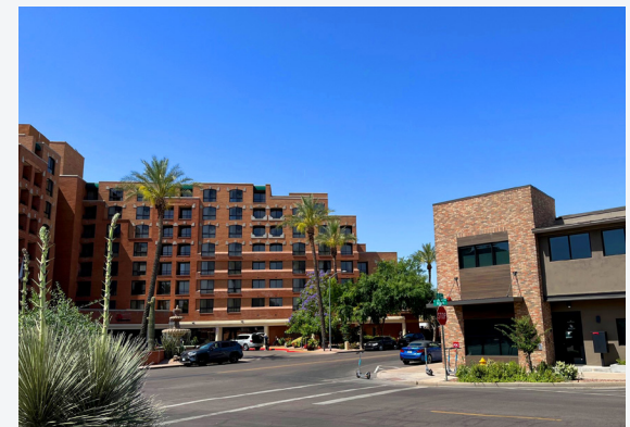
The Cavalliere blacksmith shop (left) is among the oldest buildings in Scottsdale. The office building (right) steps down in height and utilizes integrally colored materials and a gently curving masonry façade to be compatible with the thick adobe walls of the historic building.
