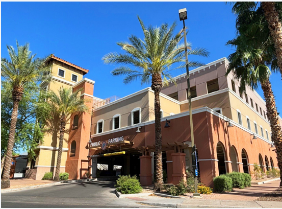
Minimize the apparent mass of a parking structure through building design and architectural features, stepbacks, and building articulation.
