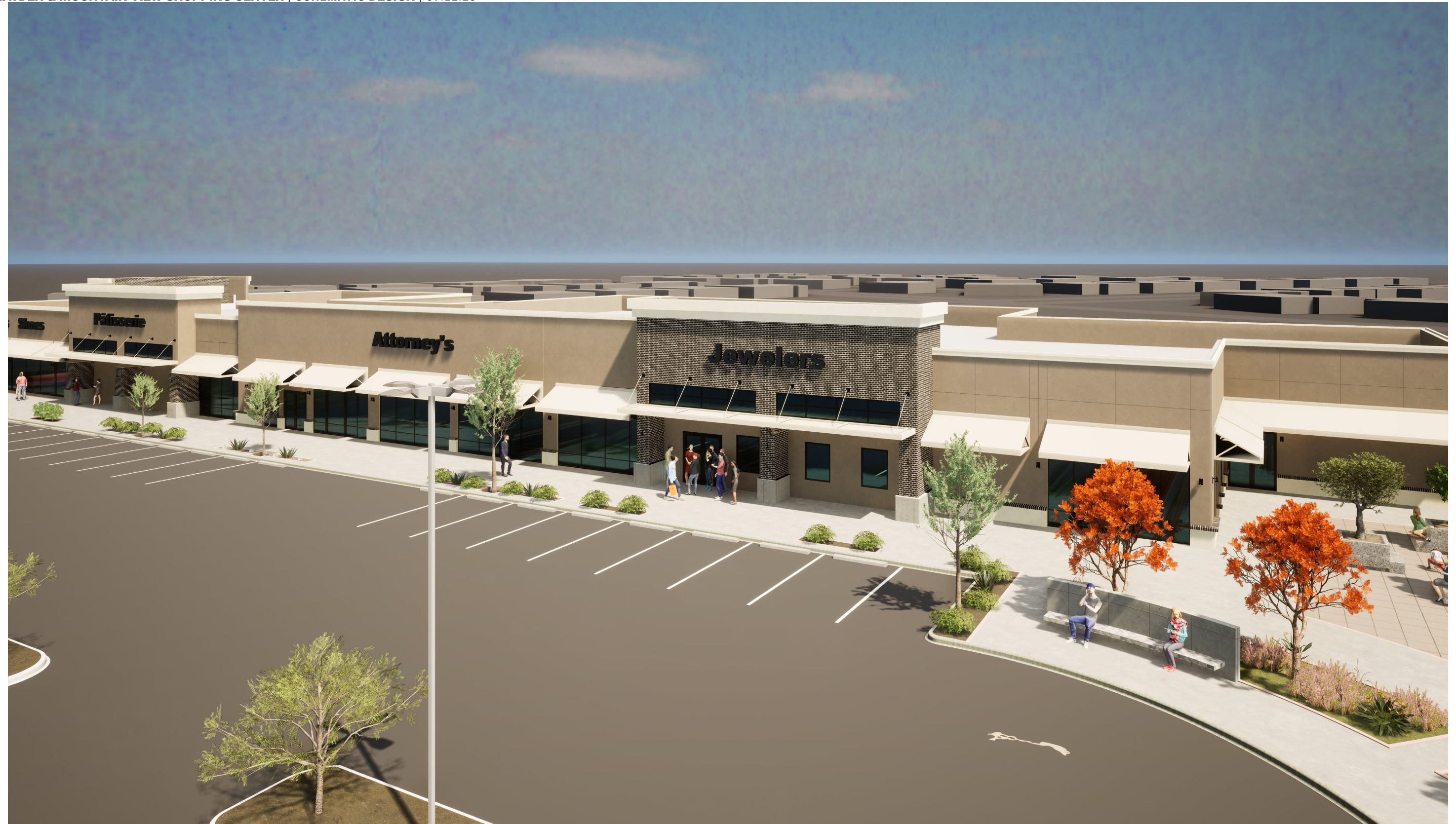
VIEW 10 BUILDING C
