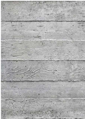
CN.1 CONCRETE, BOARD FORM LOCATION: BUILDING BASE AND GROUND LEVEL WALK-UPS FINISH: LIGHT GRAY
