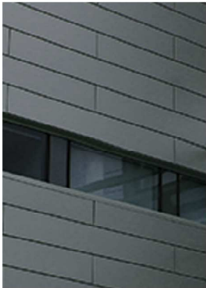
MTL.1 ALUMINUM COMPOSITE MATERIAL LOCATION: PRIMARY BUILDING CORNERS PRODUCT EXAMPLE: ALUCOBOND PLUS FINISH: MATTE - GRAY LRV: 17.77 MANUFACTURER: ALUCOBOND
