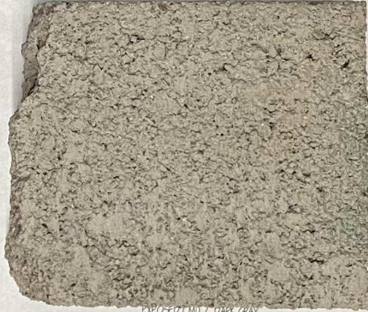
EXPOSED CMU / DARK GRAY MASONRY LOWER LEVEL WALLS
