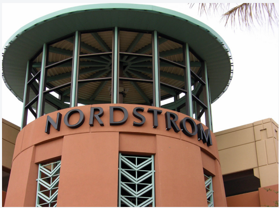
The corner of this parking garage is articulated as a stair tower giving the structure the appearance of a building.
