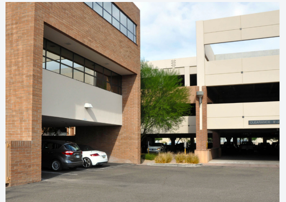
A single parking bay incorporated into the building design, and internal to the site, beneath the second floor.
