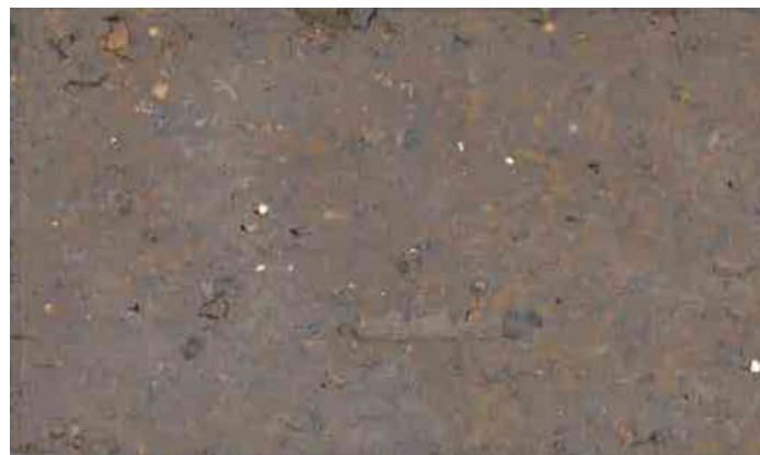
1 Bronzestone Brick Interstate Brick - Atlas Structural Brick Building/Canopy Columns
