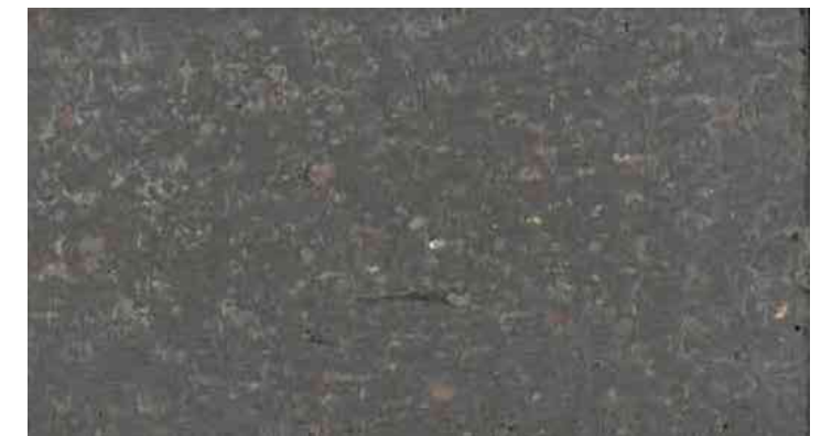
2 Midnight Brick Interstate Brick - Atlas Structural Brick Building/Canopy Columns
