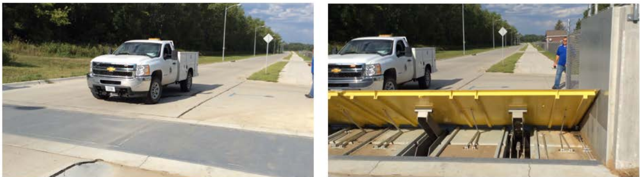
Figure 3: Floodgate in non-deployed position (left) and being mechanically deployed (right)
