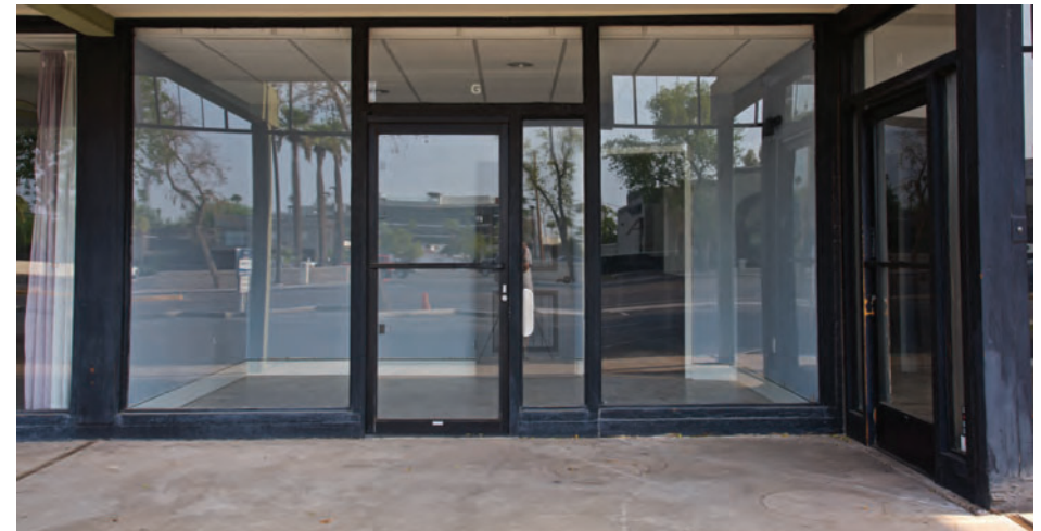
Bronze-anodized aluminum doors have replaced many of the original mill-finished aluminum doors in the wood storefronts.
