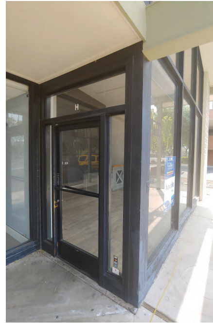
Compare loss of integrity where dark doors replace original mill-finished aluminum doors.
