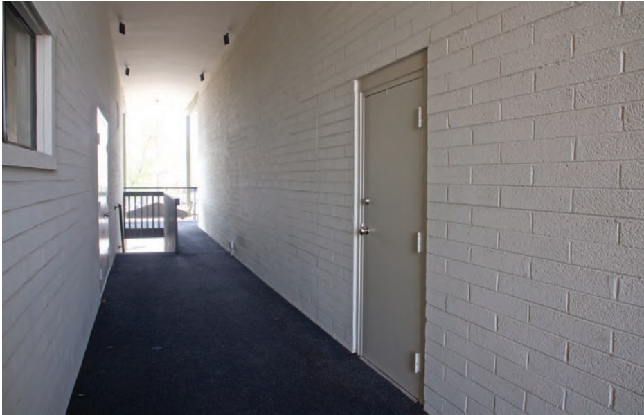
Painted gypsum board ceilings, concrete block walls, and non-historic outdoor carpeting are finishes in the second-floor breezeway. Steel doors have been relocated and added in the breezeway.
