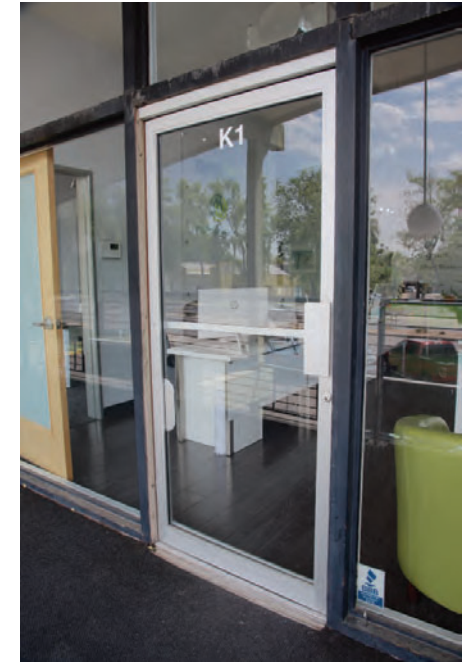
Compare loss of integrity where dark doors replace original mill-finished aluminum doors.
