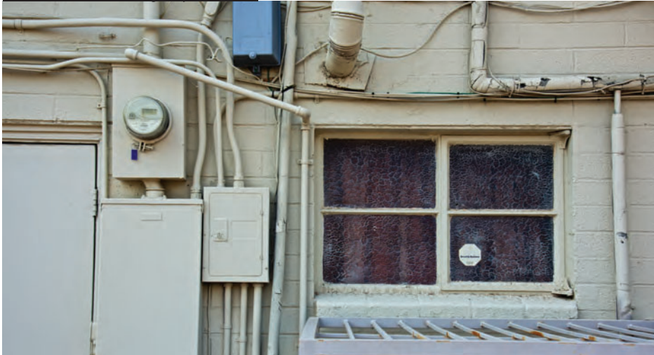
many generations of electrical system modifications are evident on the rear elevation
