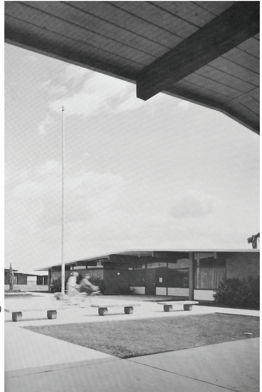
1959 Hohokam Elementary School
