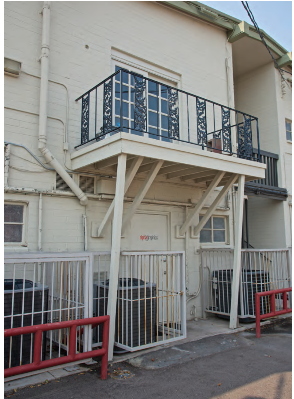
A remnant of the original cast iron balcony guardrails survives at the rear balcony.
