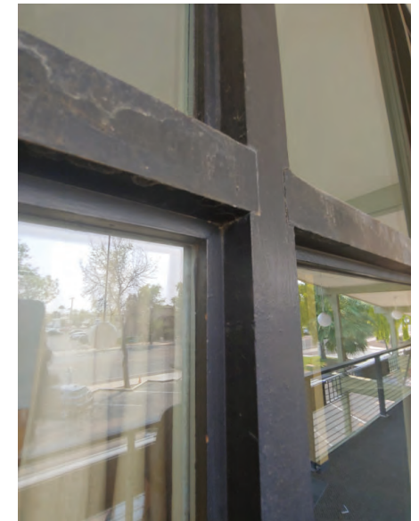
Expert workmanship survives in the joinery of the original wood storefronts.
