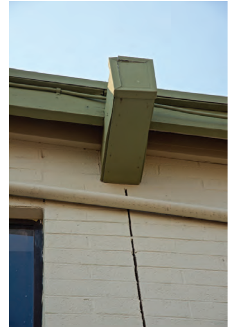
The economical laminated beams supporting the roof and second floor have been sheathed to protect from weather and to enhance their appearance.
